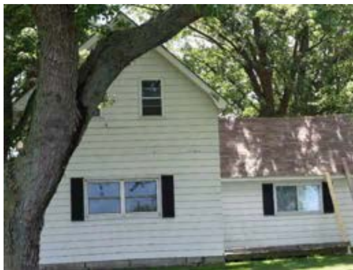
North (front) façade of house on property
