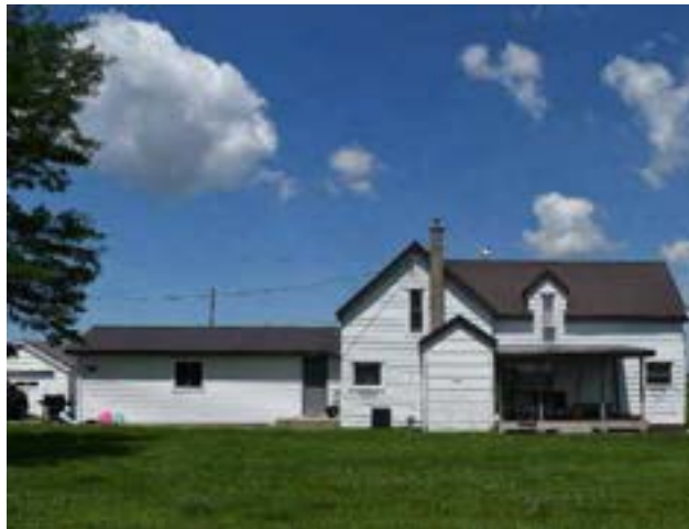
South (front) façade of house on property
