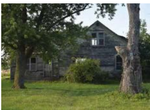
South (front) façade of house on property
