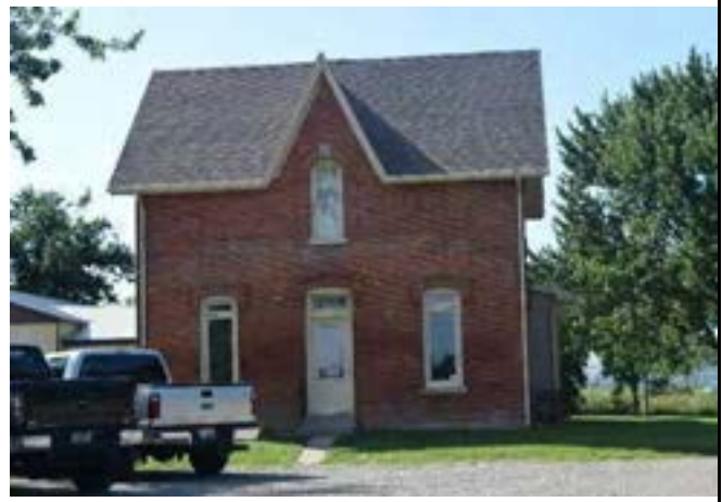
South (front) façade of house on property
