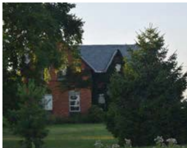
South (front) façade of house on property
