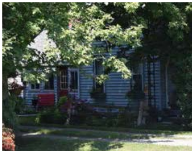
East (front) façade and south wall of house on property
