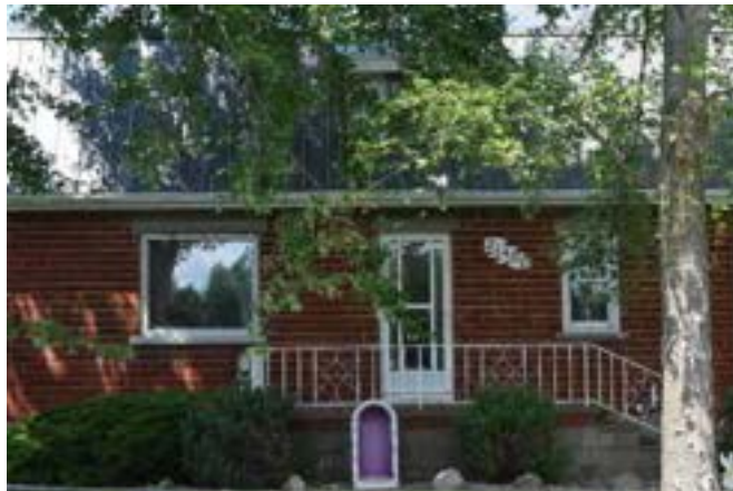
South (front) façade of house on property
