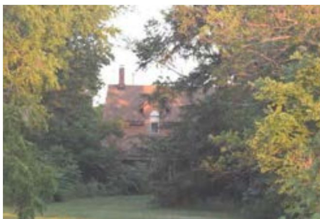
North (front) façade of house on property
