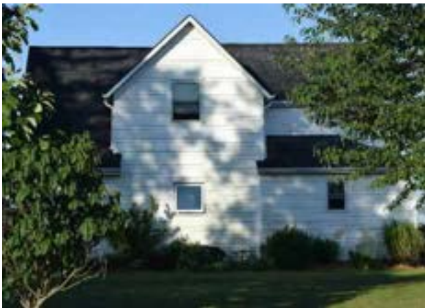
East (front) façade of house on property
