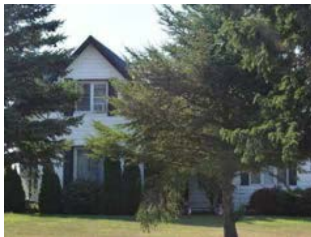
North (front) façade of house on property
