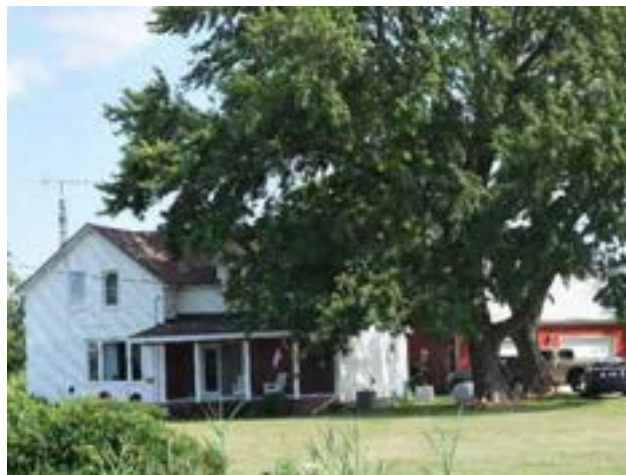
North (front) façade of house on property
