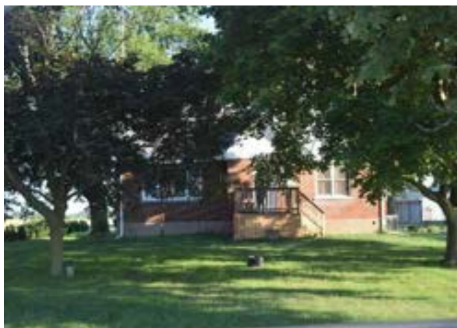
South (front) façade of house on property
