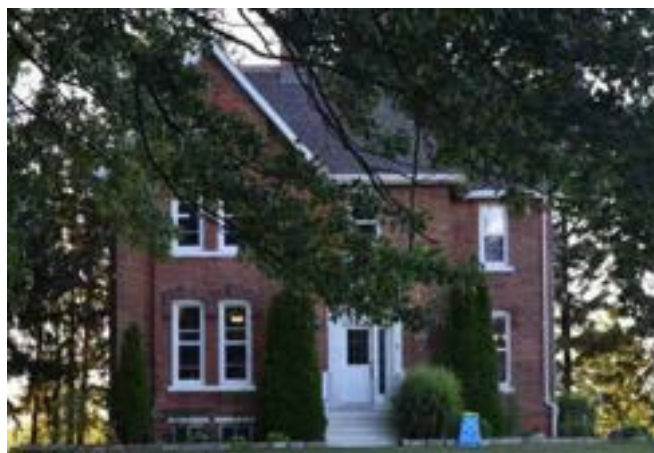
South (front) façade of house on property
