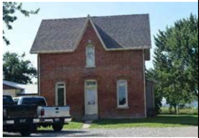
South (front) façade of house on property
