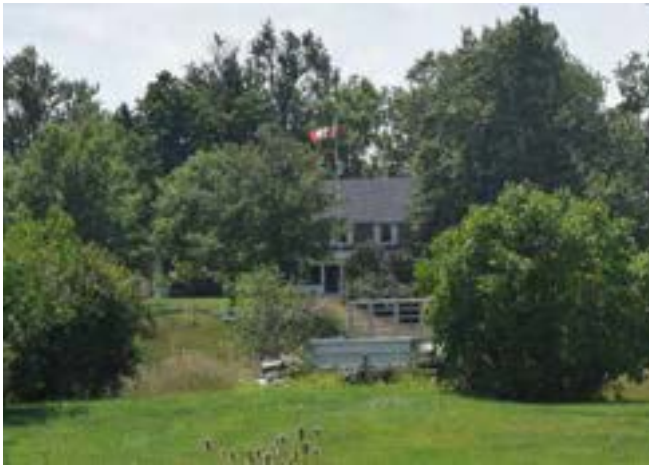
North (front) façade of house on property
