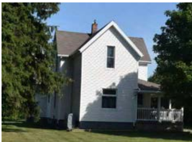
South (front) façade of house on property
