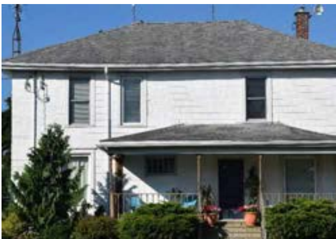
East (front) façade of house on property
