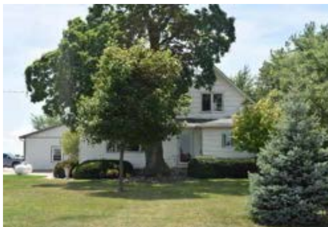
East (front) façade of house on property
