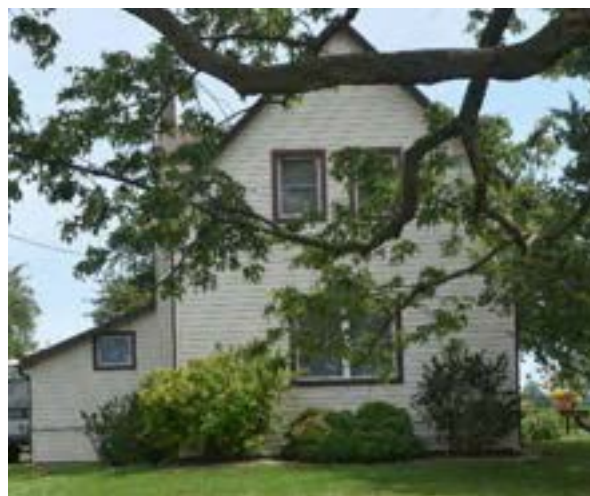
North (front) façade of house on property
