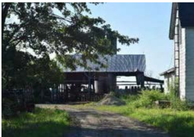
Associated open air barn on property, looking north from Seventh Line East
