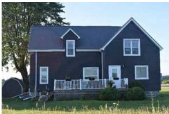
North (front) façade of house on property
