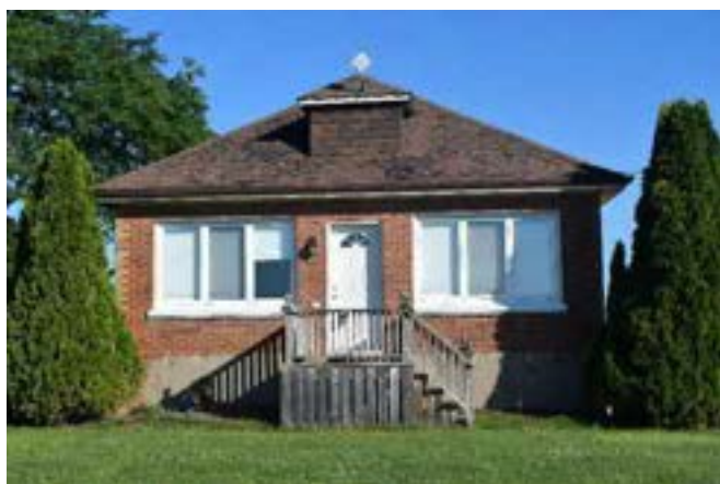
South (front) façade of house on property
