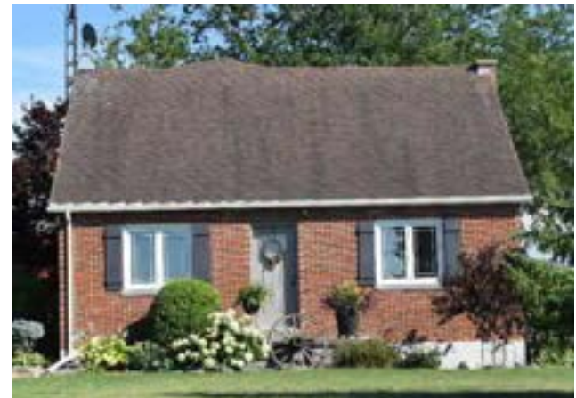
North (front) façade of house on property
