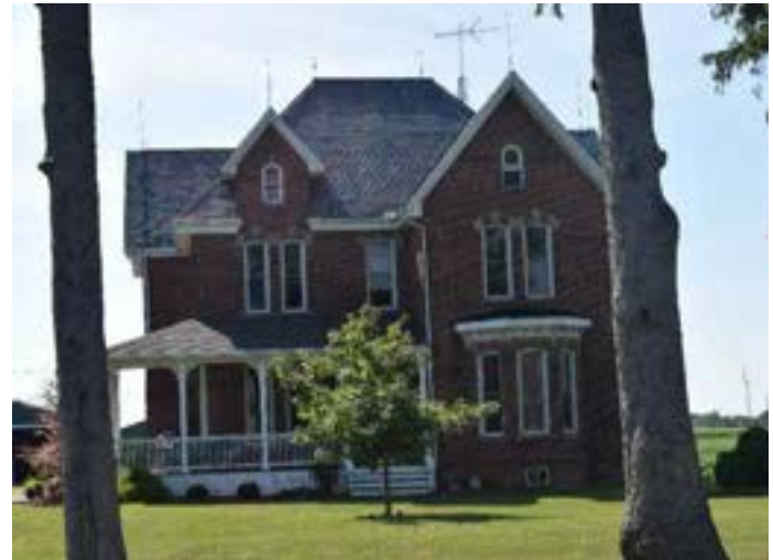
North (front) façade of house on property
