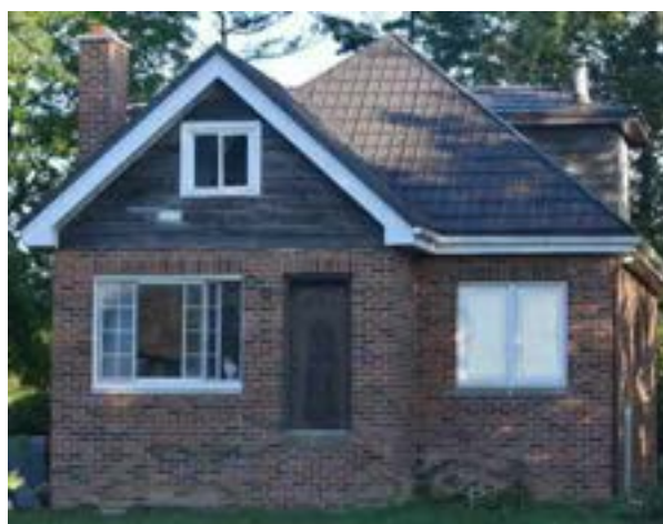
South (front) façade of house on property
