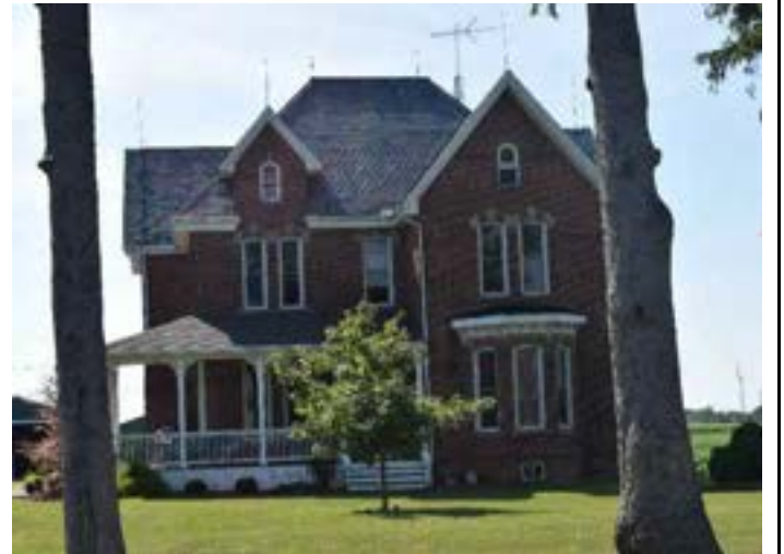
North (front) façade of house on property
