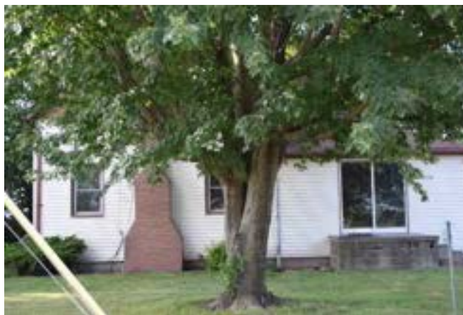
South (front) façade of house on property
