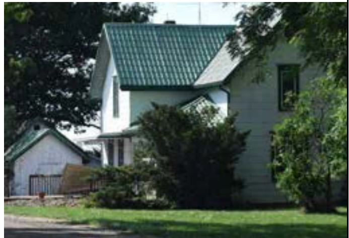
North (front) façade of house on property
