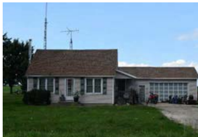
South (front) façade of house on property
