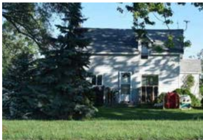
South (front) façade of house on property
