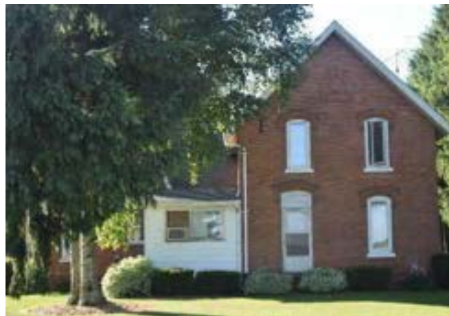
North (front) façade of house on property
