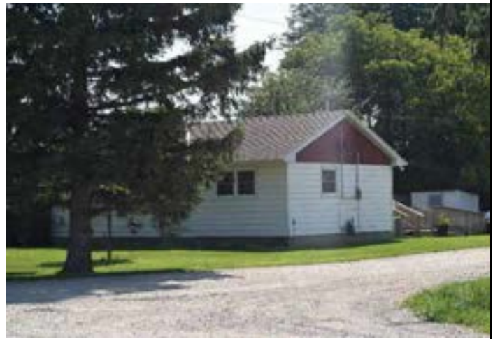
Associated house/ structure on property, looking southeast from 6 Line East
