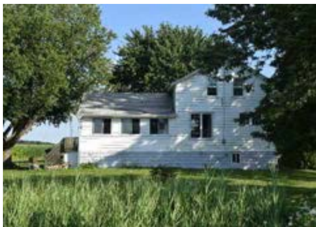
South (front) façade of house on property
