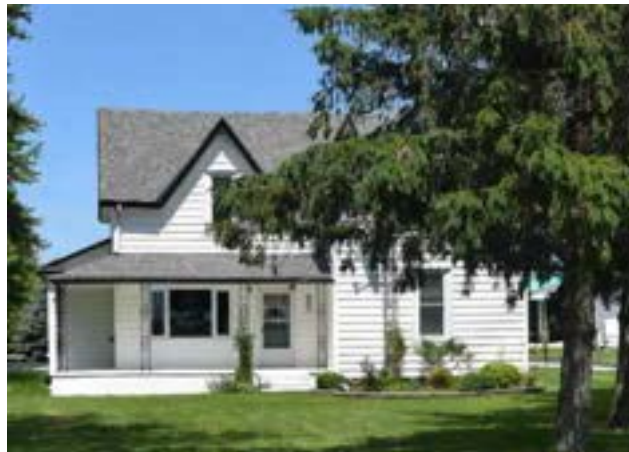
South (front) façade of house on property
