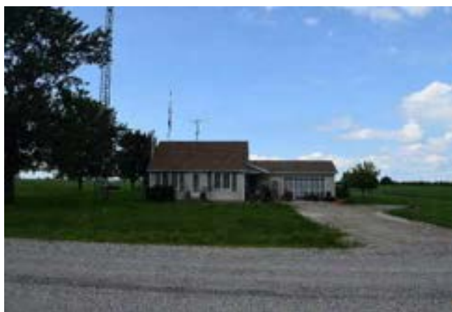
Property lot, looking north from Morris Road
