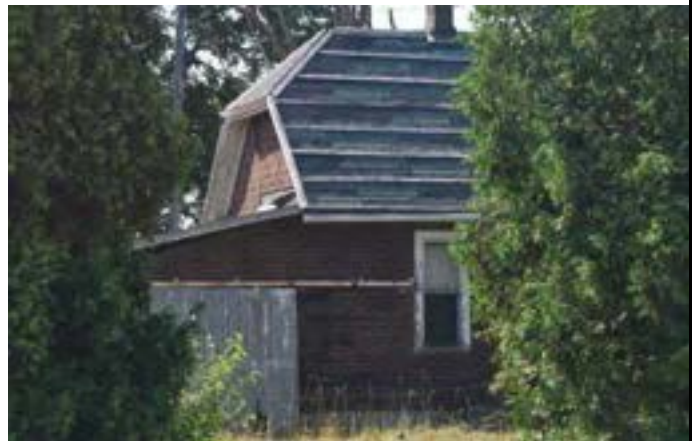
Associated structure on property, looking south from 8 Line
