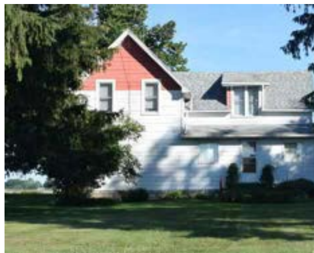
South (front) façade of house on property
