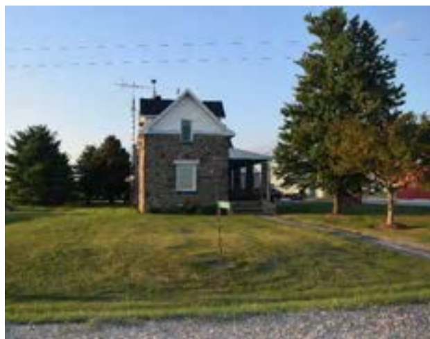
South (front) façade of house on property
