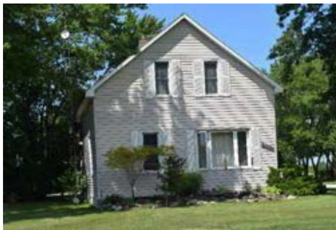
South (front) façade of house on property
