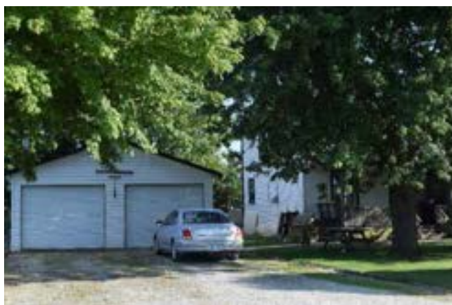
North (front) façade of house on property
