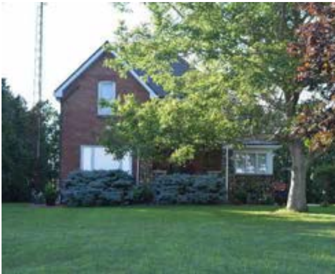
Property lot, looking northwest from 6 Line
