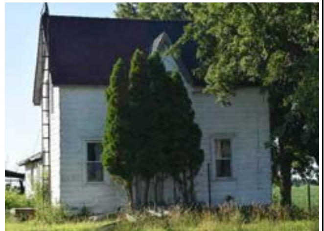
South (front) façade of house on property
