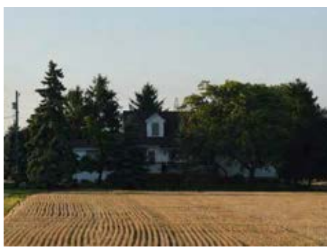
South (front) façade of house on property
