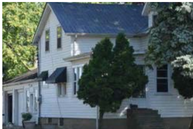
West (front) façade and south wall of house on property
