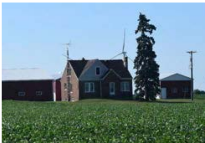
North (front) façade of house on property
