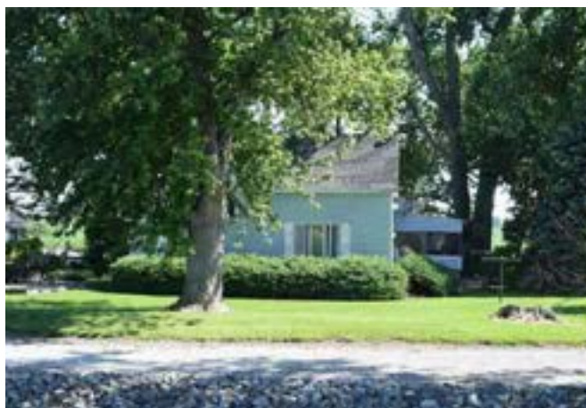
West wall of house on property
