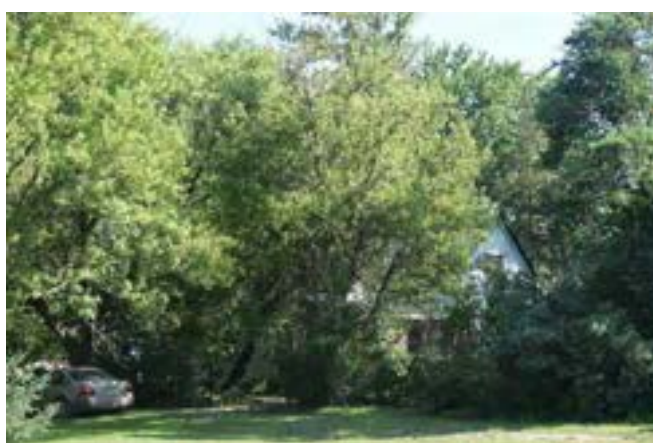
South (front) façade of house on property
