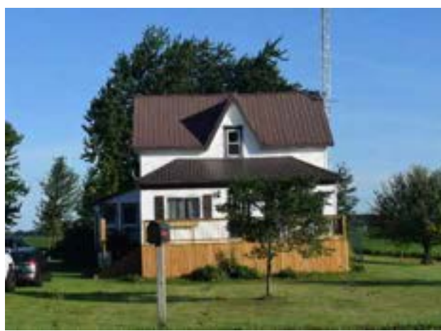
South (front) façade of house on property
