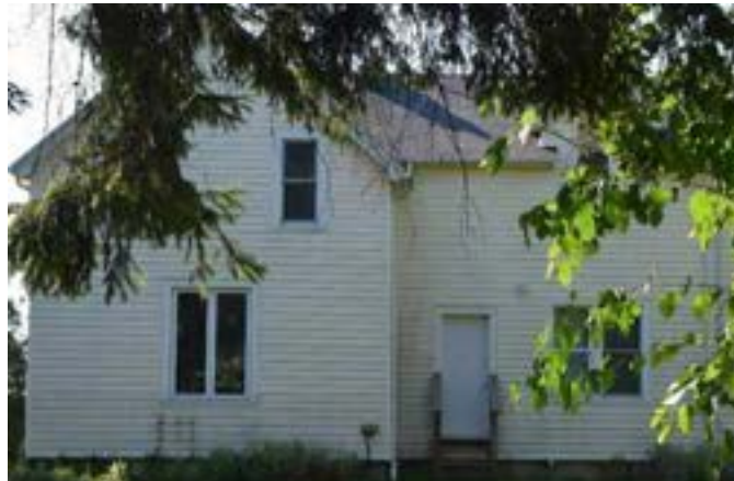
South (front) façade of house on property
