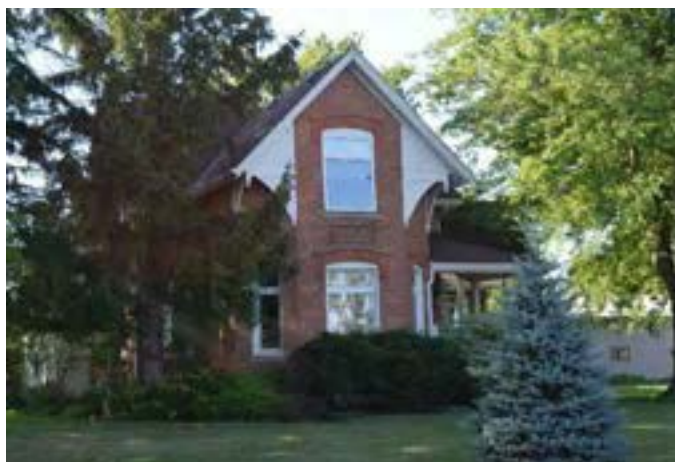
South (front) façade of house on property
