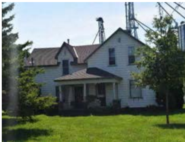
North (front) façade of house on property
