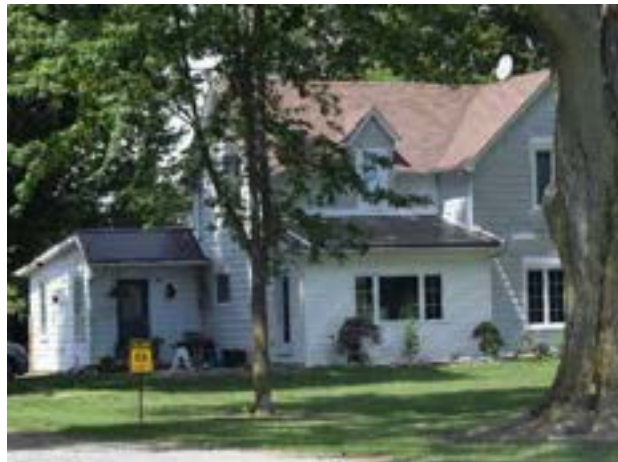
South (front) façade of house on property
