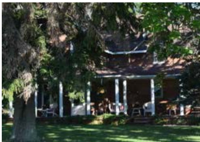
South (front) façade of house on property
