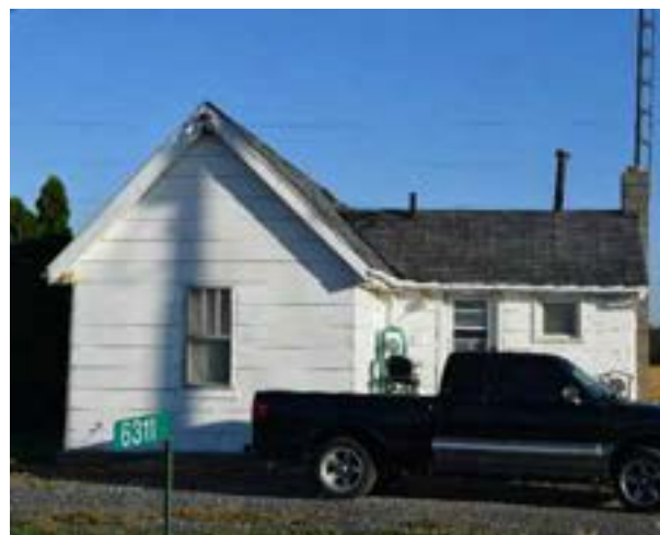
South (front) façade of house on property
