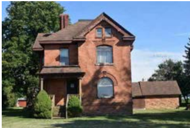
North (front) façade of house on property
