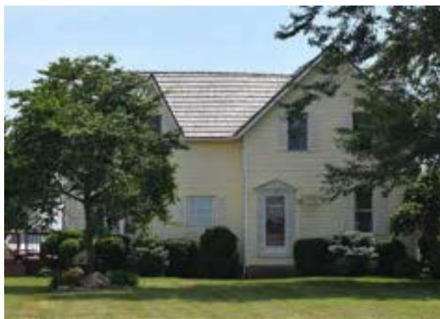
North (front) façade of house on property
