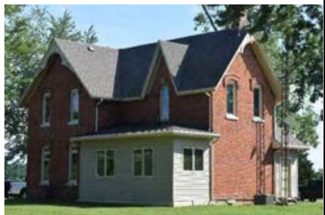
North façade and east wall of house on property
