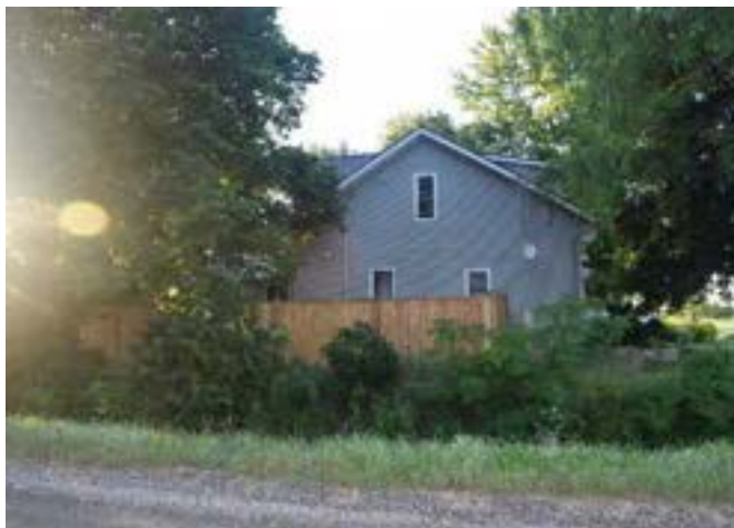
North wall of house on property
