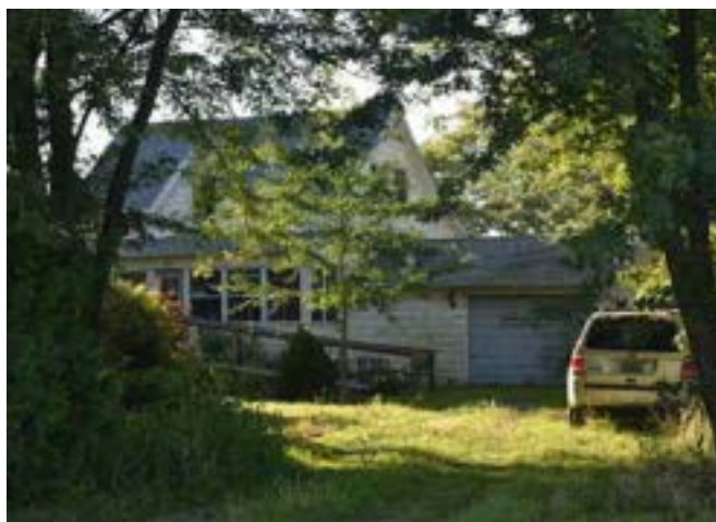
North (front) façade of house on property
