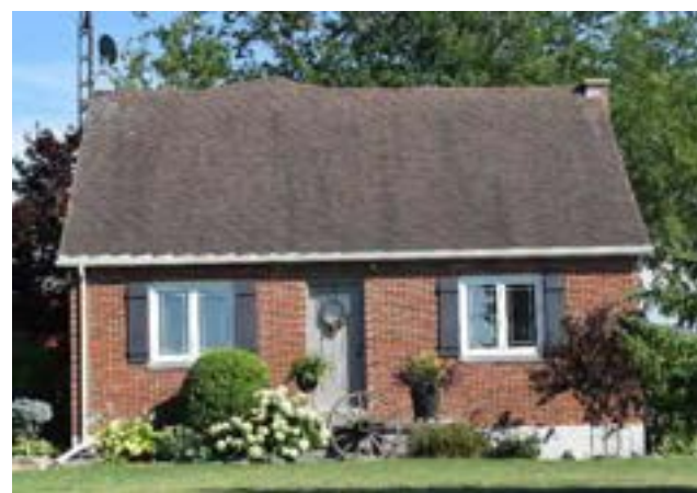
North (front) façade of house on property
