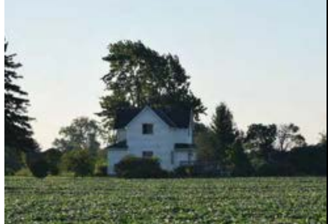
North façade of house on property
