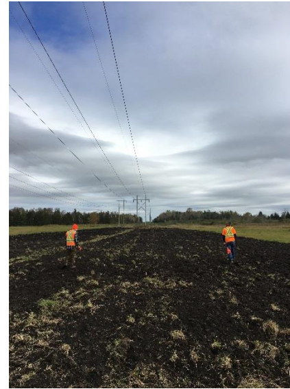
Photo 18: Crew at work at PIN 583540024, facing east.
