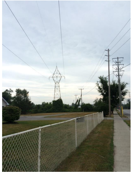
Photo 30: Hydro corridor through residential property; view northwest
