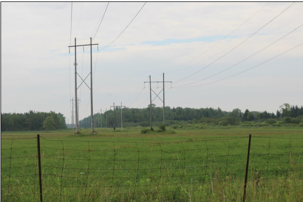
Figure 14: View of hydro corridor from Grenfel Road
