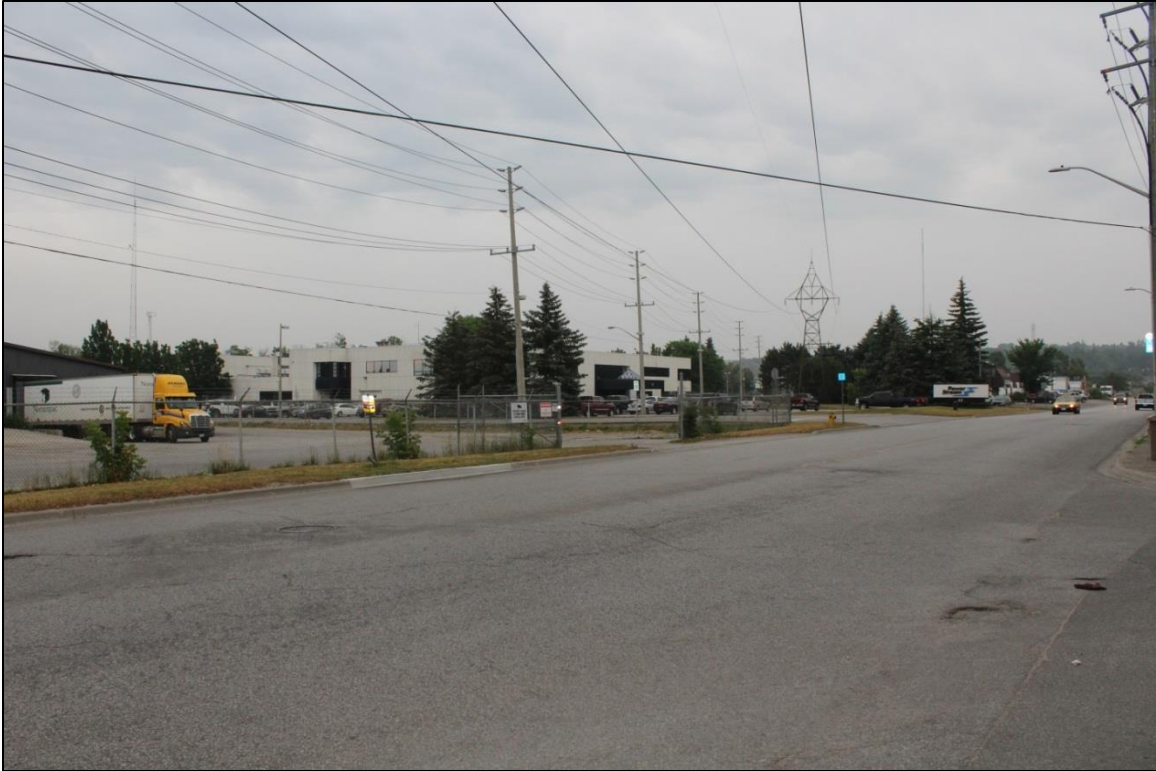
Figure 1: View to south east of existing hydro corridor along Patterson Avenue
