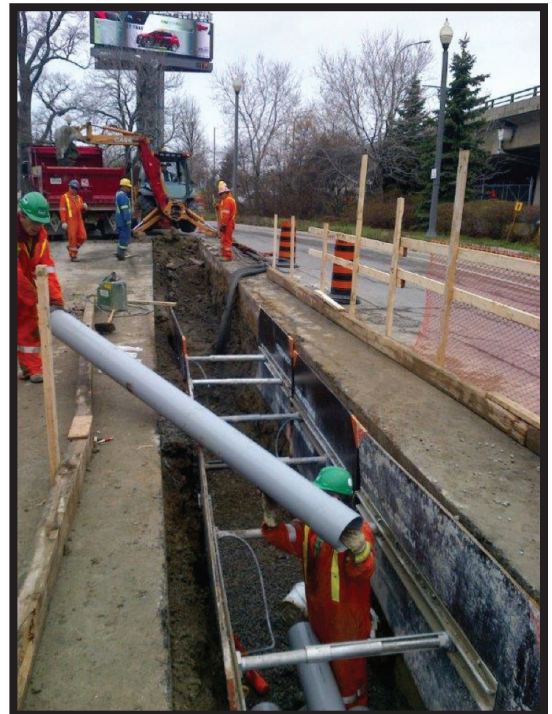
Example of duct bank installation used to house new cables
