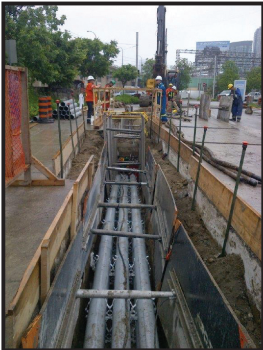
Example of open excavation construction
