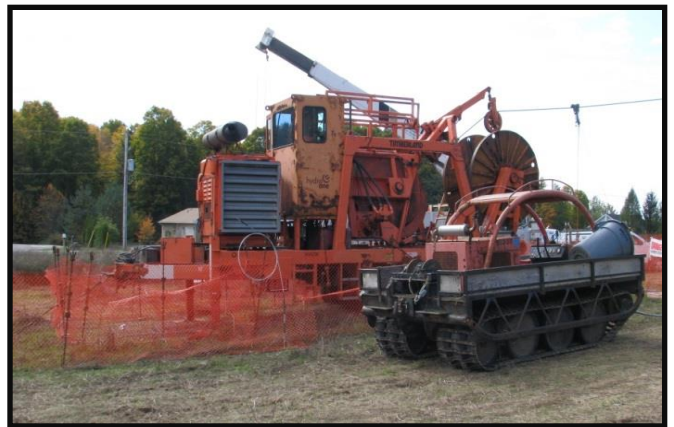
Set up laydown area
