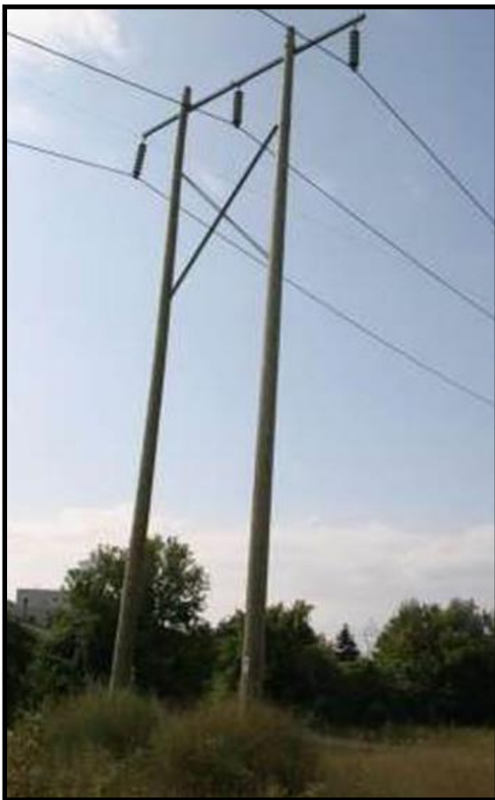
Existing 2-pole structure
