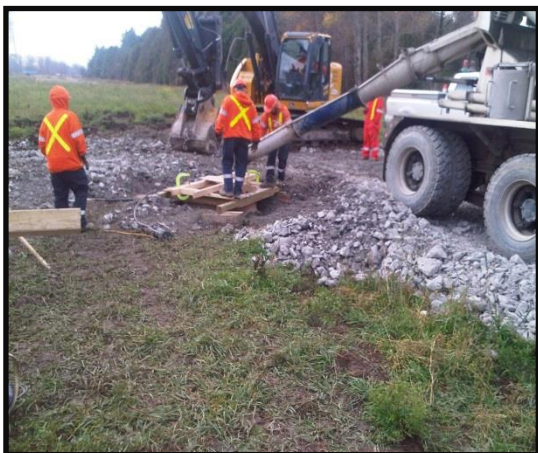
Pouring concrete for tower foundation
