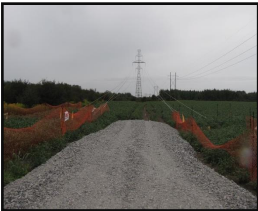
Temporary access road
