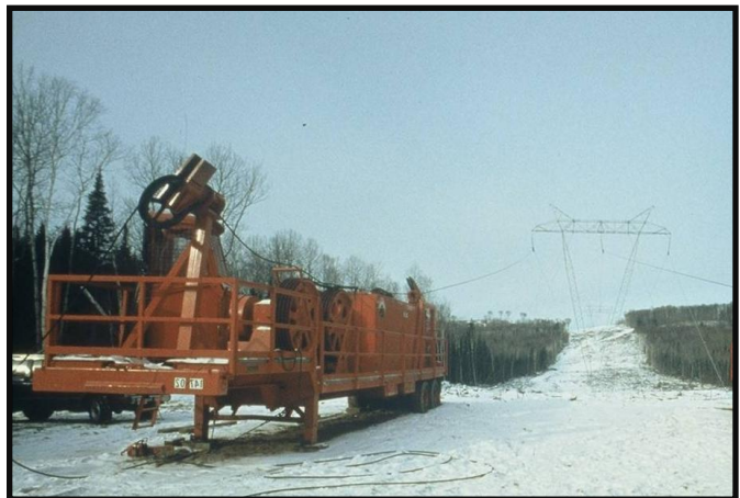
Pulling new conductor into position
