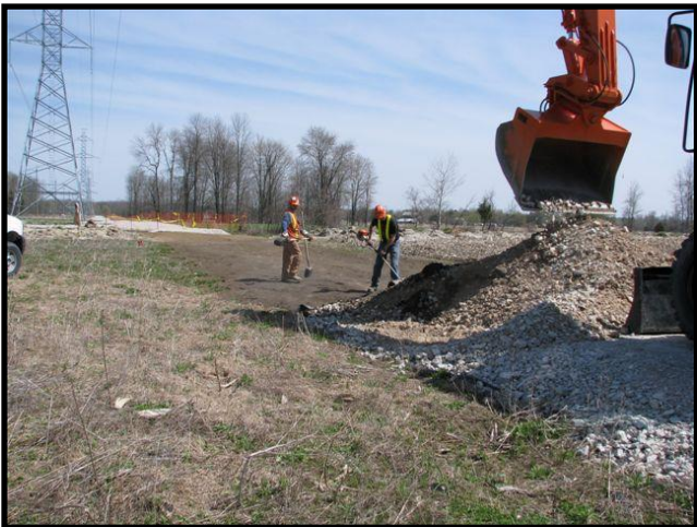
Remove temporary access road
