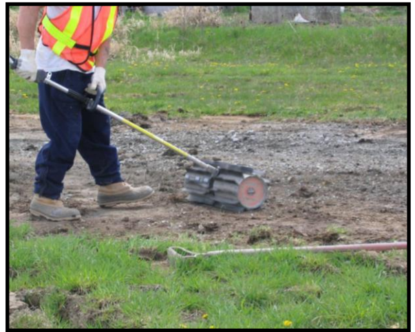
Remove remaining crushed stone
