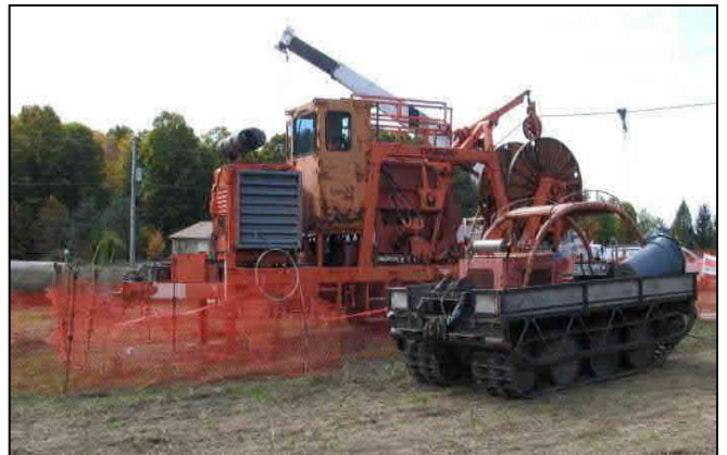
Set up laydown area
