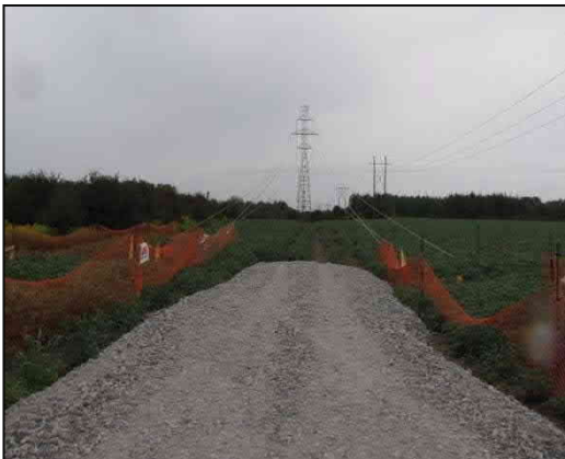
Temporary access road
