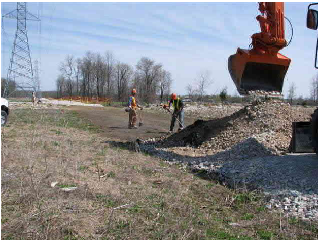
Remove temporary access road
