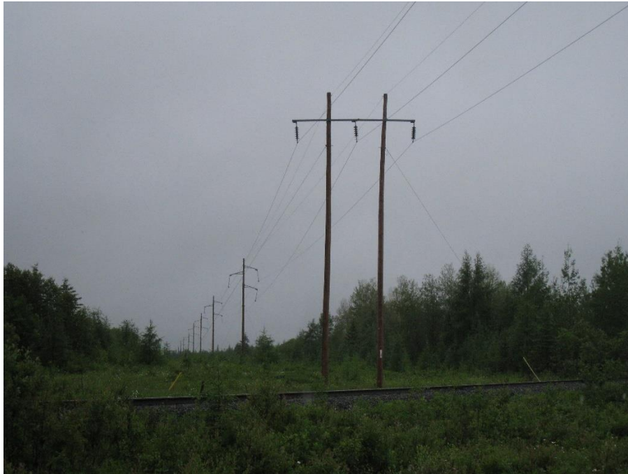
Figure 1: Typical Suspension H Frame Wood Structure
