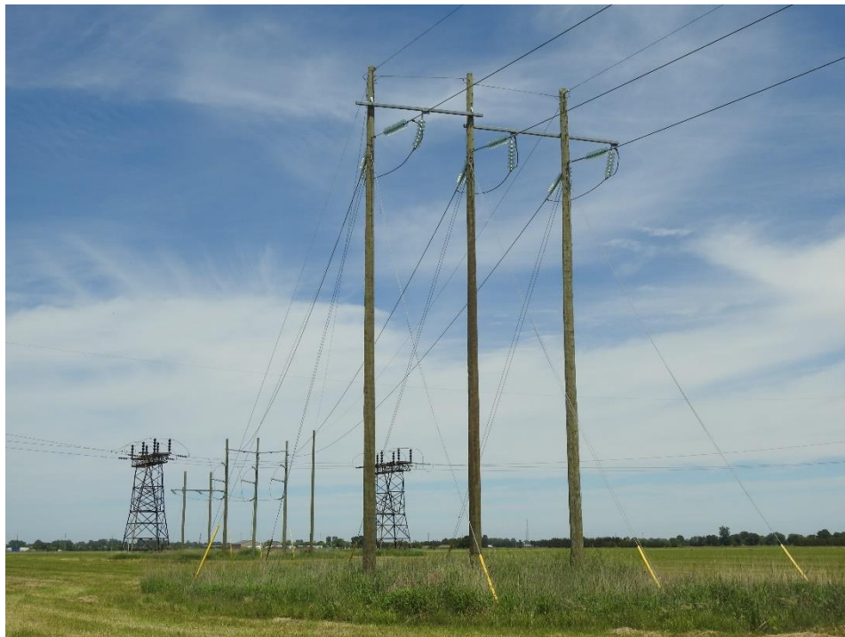
Figure 2: Typical 3-Pole Deadend Wood Structure
