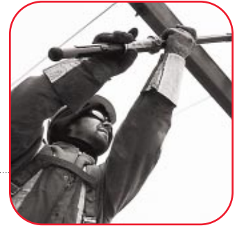
Wood pole replacement in Allanburg
