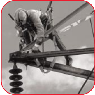
Scheduled feather (transmission tower arms) replacement in Mississauga
