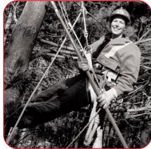
Clearing branches away from power lines helps to ensure system reliability. Pictured is Kim Meeker, Regional Maintainer – Forestry.
