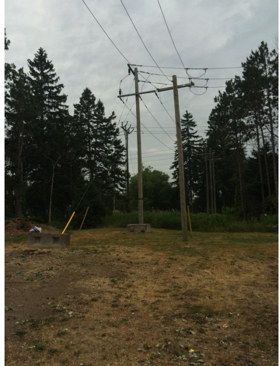
Photo 2: Cleared area southwest of existing transmission station; view west
