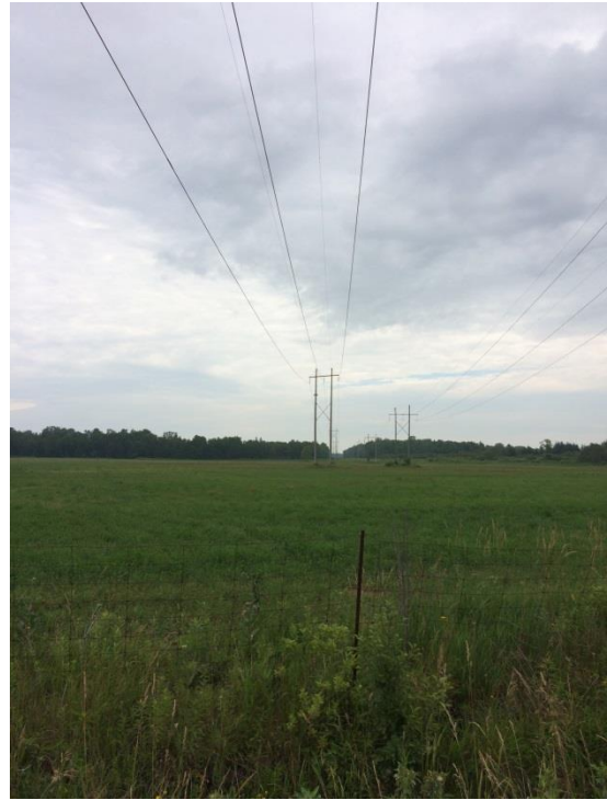
Photo 26: Hydro corridor through active agricultural field; view east
