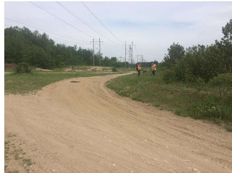
Photo 24: Crew at work at PIN 583530154, facing north.
