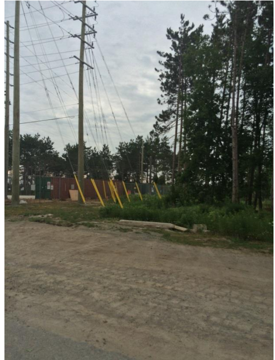
Photo 4: Barrie Transmission Station, disturbance from hydro tower; view northeast
