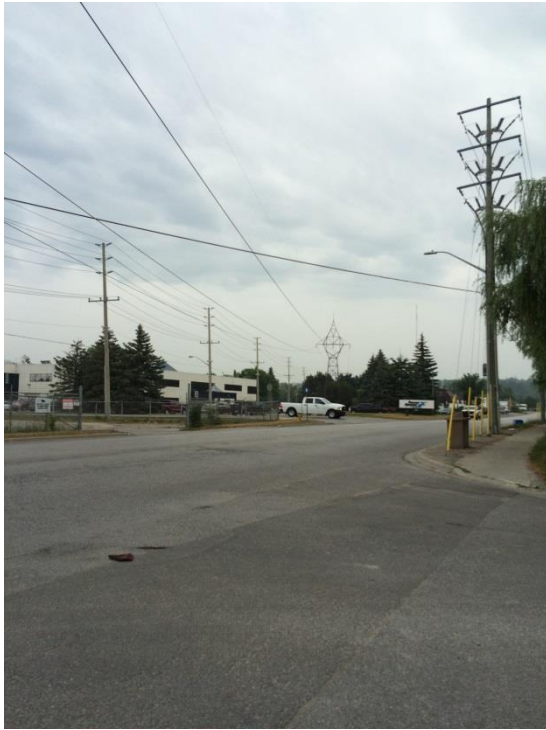
Photo 29: Hydro corridor through residential and industrial locations; view southeast
