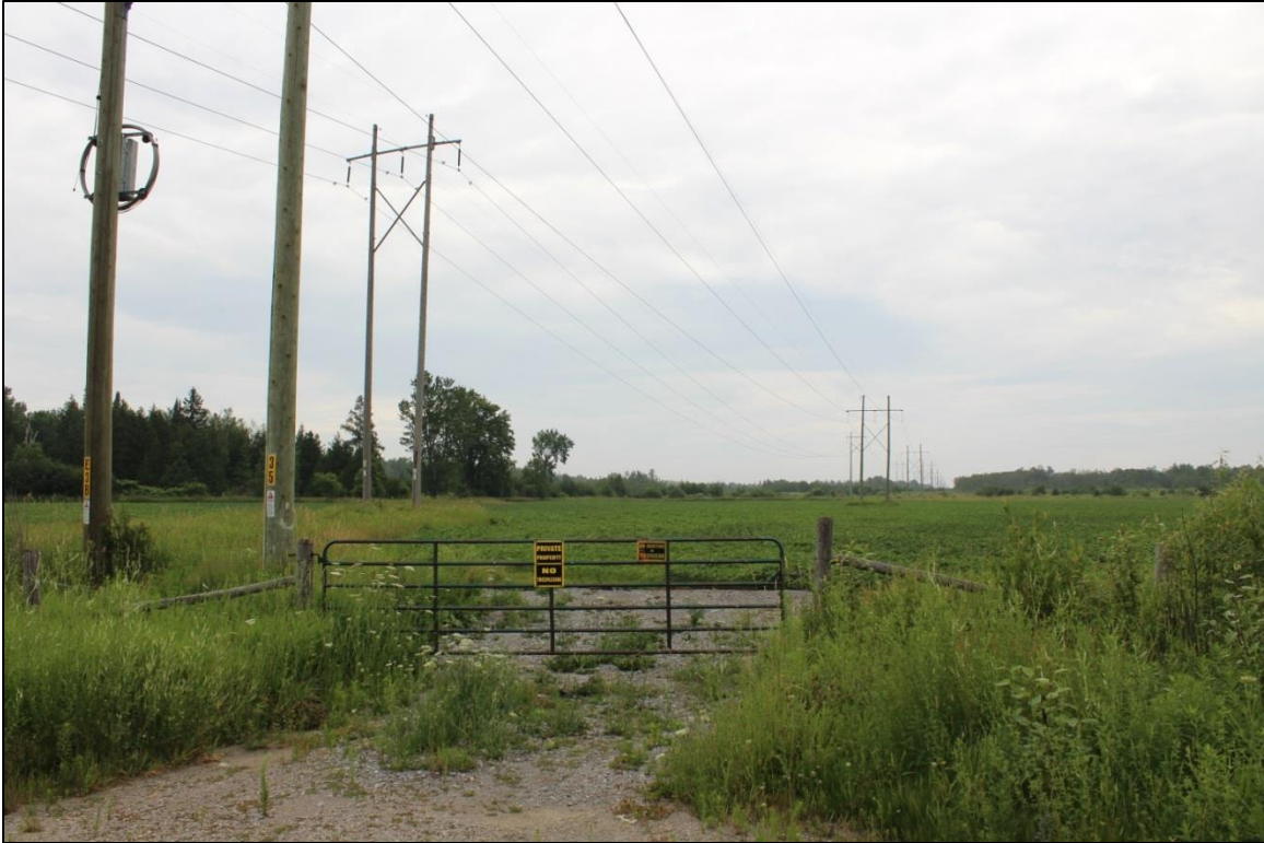
Figure 13: View to east of hydro corridor from George Johnston Road
