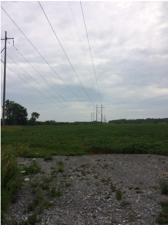
Photo 23: Hydro corridor through active agricultural field; view east
