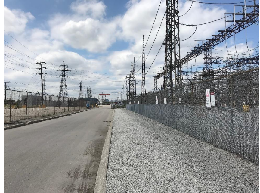
Plate 14: View from Kipling Avenue; Area is disturbed, no potential
