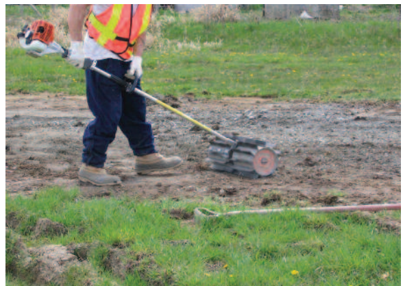
Removing remaining crushed stone
