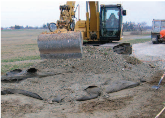
Removing temporary access road
