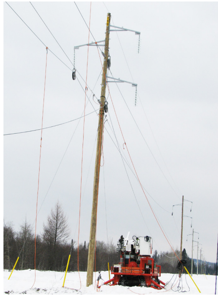
Stringing on a pole
