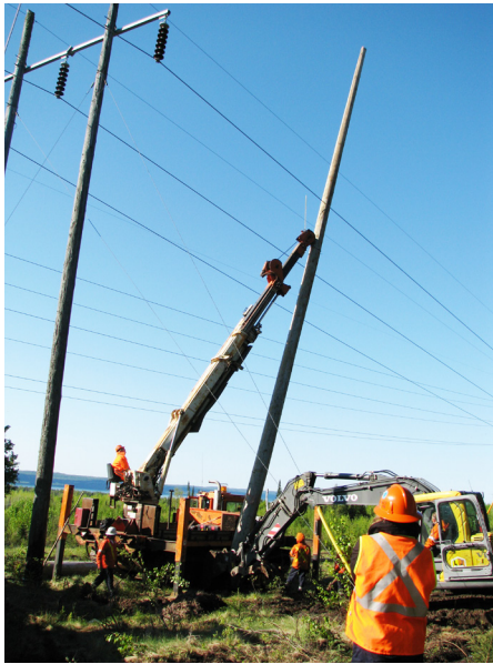
Pulling new wire into position
