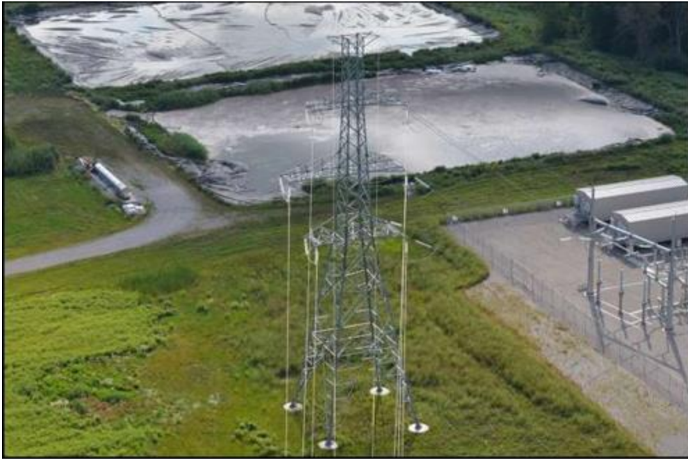
Figure 1-7: Example of a Typical Line Tap Structure
