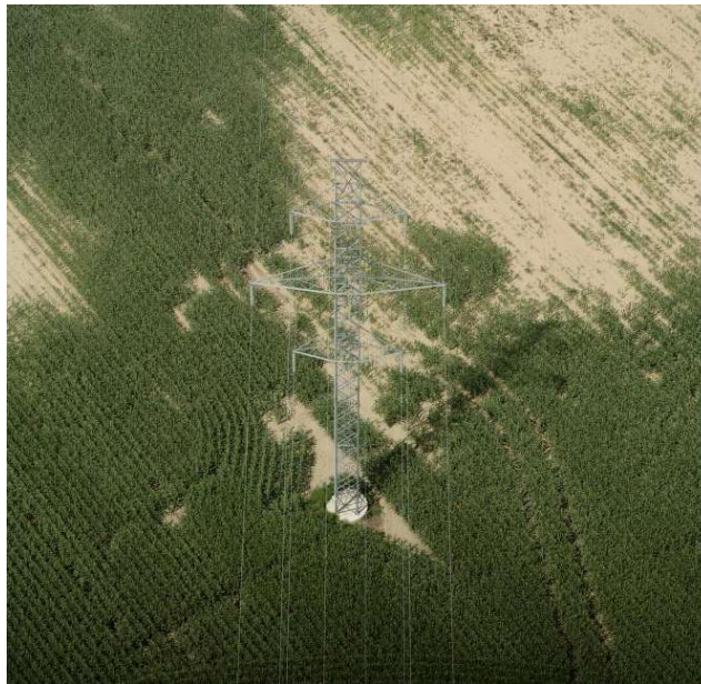
Figure 1-6: Example of a Proposed Transmission Tower
