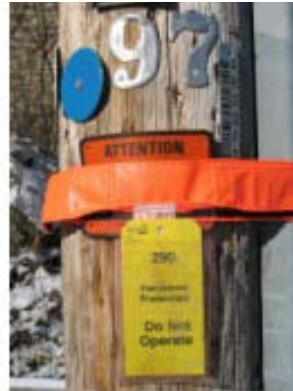
Figure B: Red Tag Holder for Hydro One Poles with Hazardous Conditions
