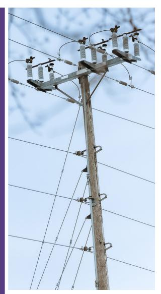
Overhead gang-operated disconnect switches on our distribution poles to help improve grid reliability.
