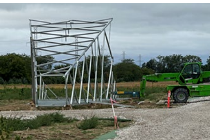
Photo of an access road and tower being assembled in Chatham
