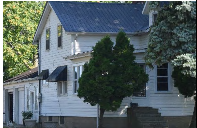
West (front) façade and south wall of house on property
