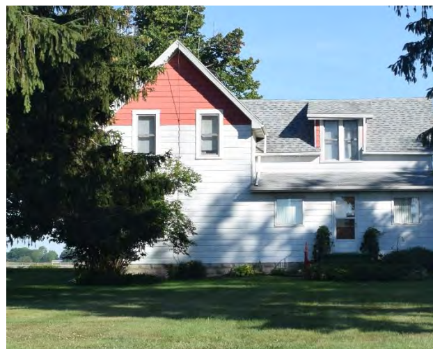
South (front) façade of house on property
