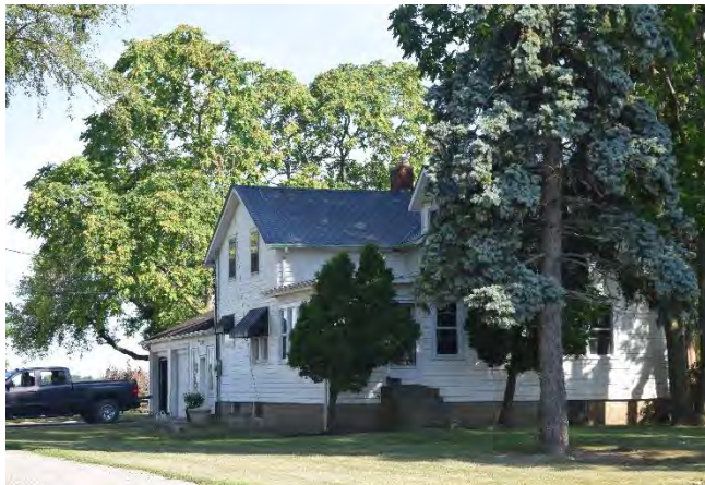
Property lot, looking northwest from 9 Line
