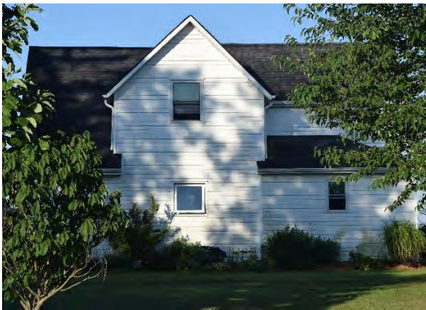
East (front) façade of house on property
