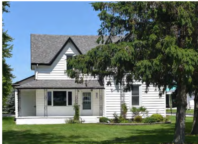
South (front) façade of house on property
