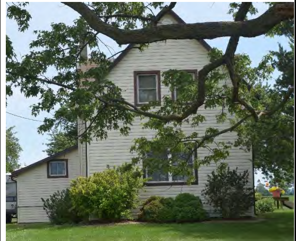
North (front) façade of house on property
