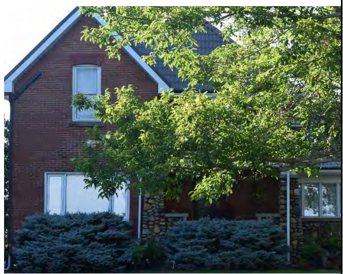
South (front) façade of house on property
