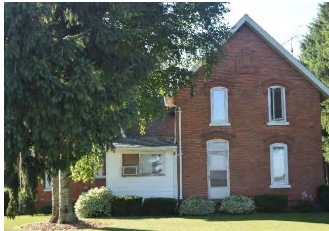
North (front) façade of house on property
