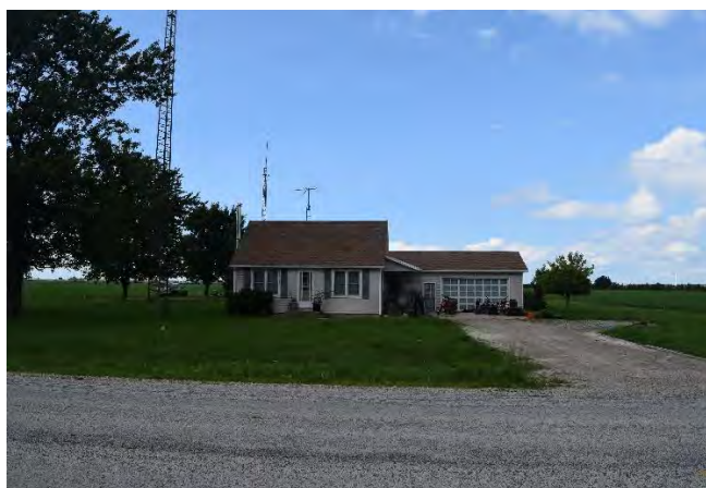
Property lot, looking north from Morris Road
