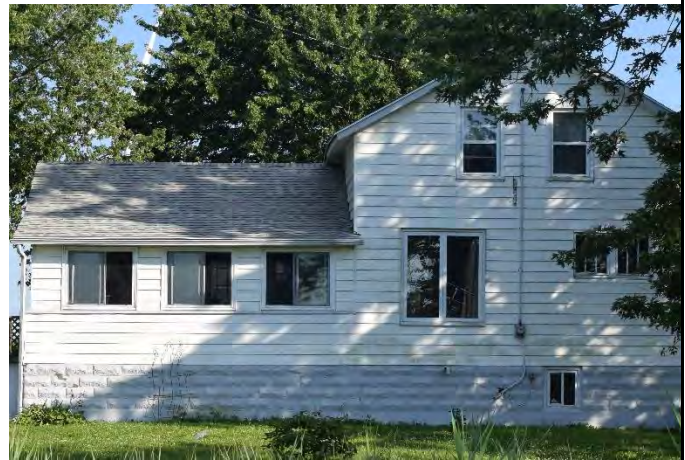
Associated barn and outbuildings on property, looking north from South Middle Road
