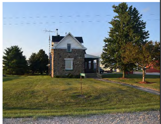
South (front) façade of house on property
