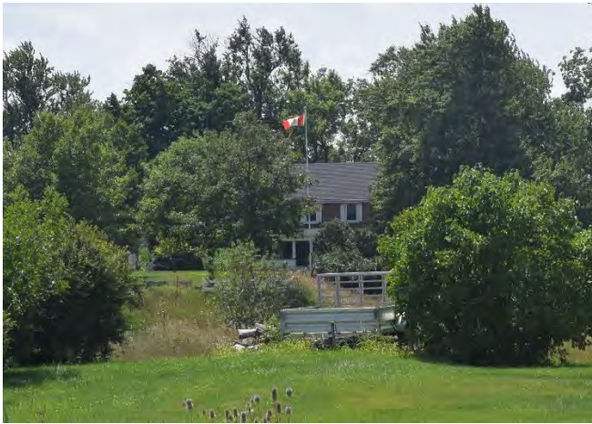
North (front) façade of house on property
