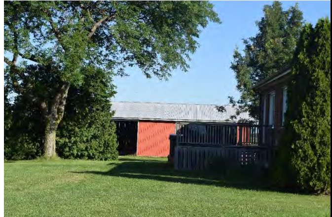
Associated barn on property, looking north from 3 Line
