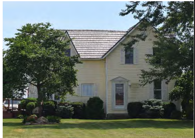
North (front) façade of house on property
