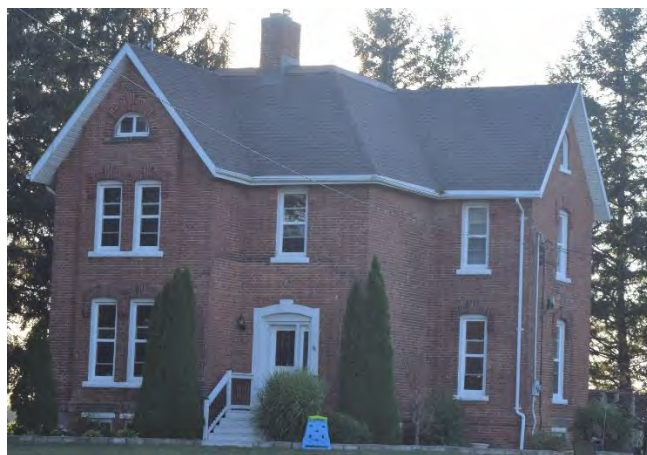
South (front) façade and west wall of house on property
