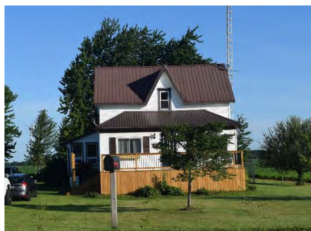
South (front) façade of house on property
