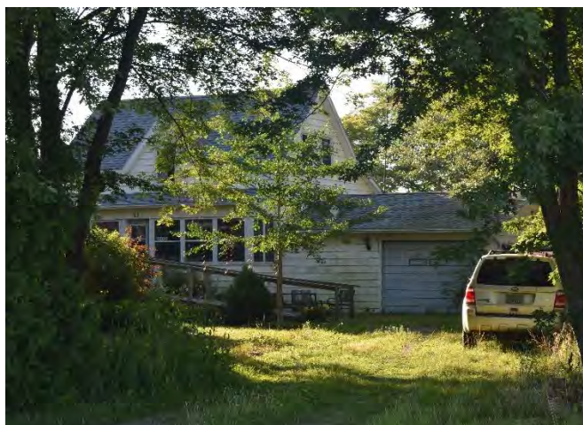
North (front) façade of house on property
