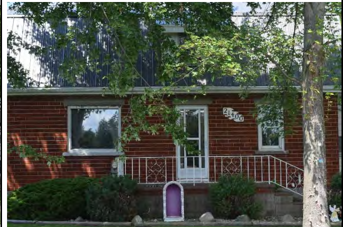
South (front) façade of house on property
