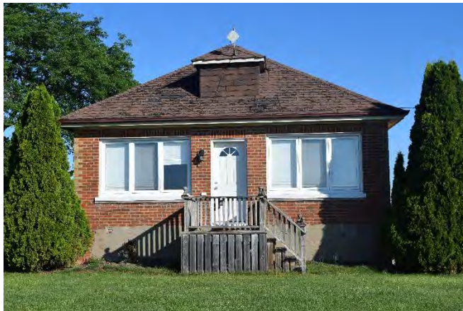
South (front) façade of house on property
