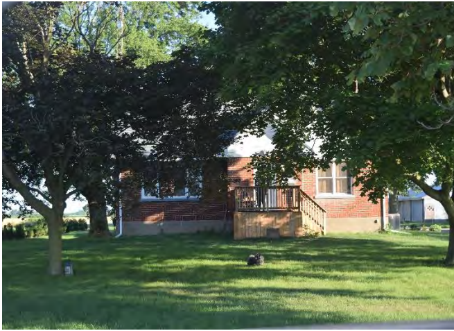
South (front) façade of house on property
