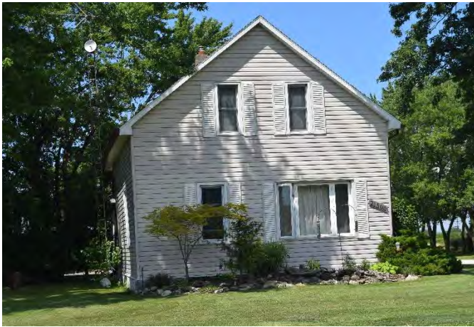
South (front) façade of house on property
