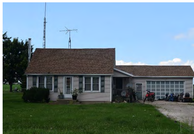
South (front) façade of house on property
