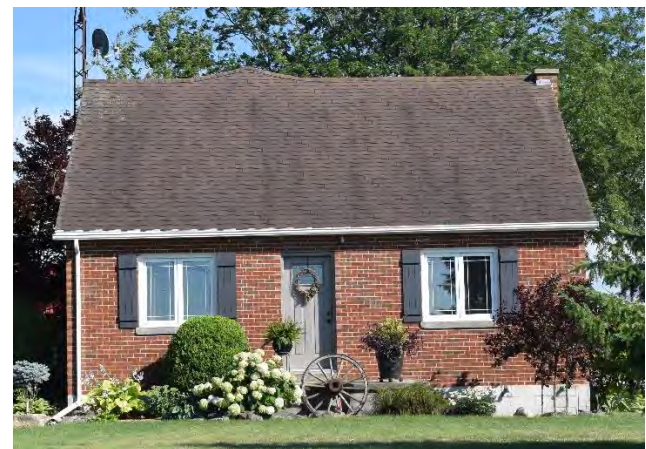
North (front) façade of house on property
