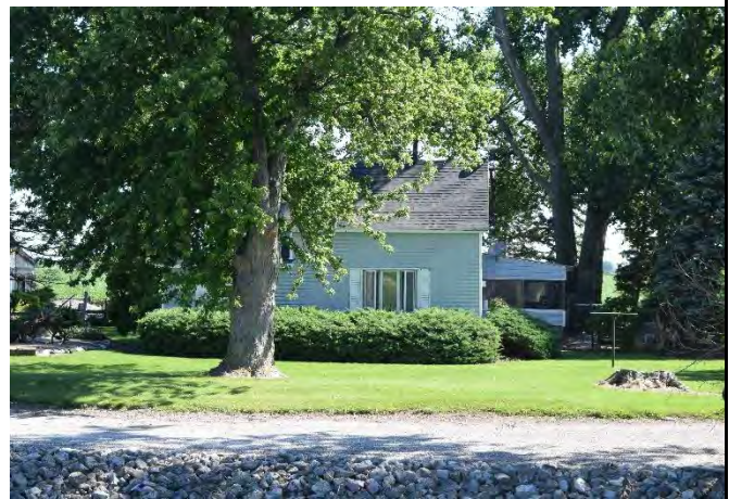
West wall of house on property
