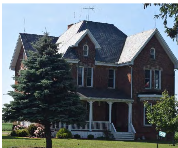
North (front) façade and east wall of house on property
