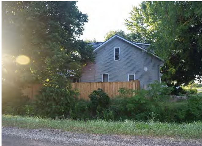
North wall of house on property
