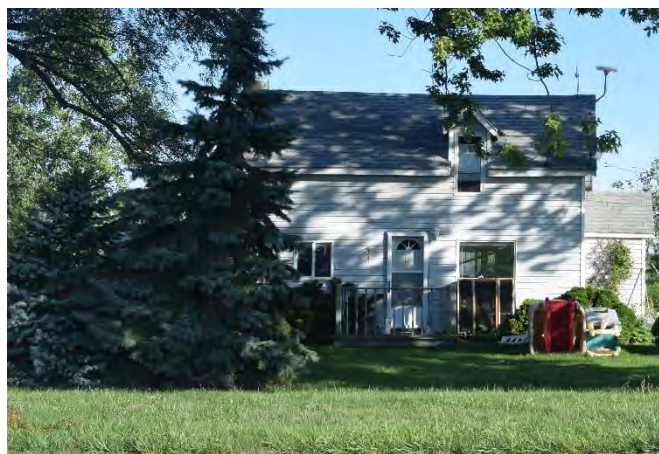
South (front) façade of house on property
