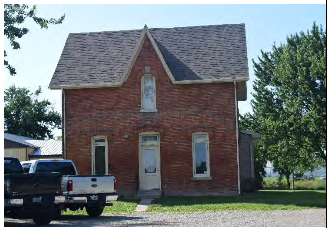
South (front) façade of house on property
