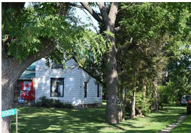
South (front) façade and east wall of house on property
