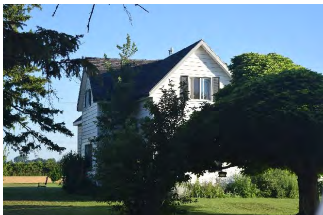
South (front) façade and west wall of house on property
