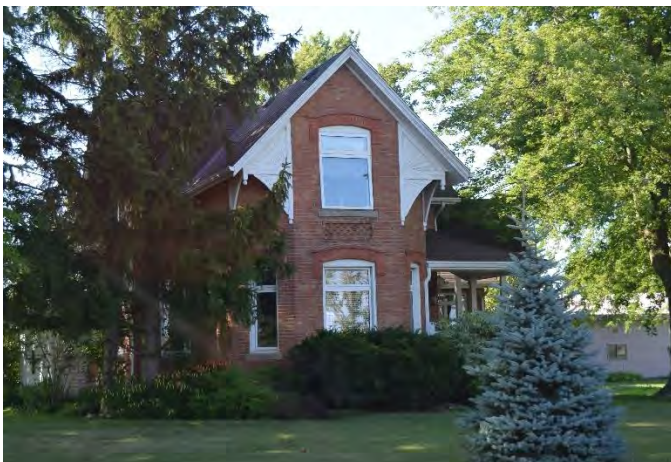
South (front) façade of house on property
