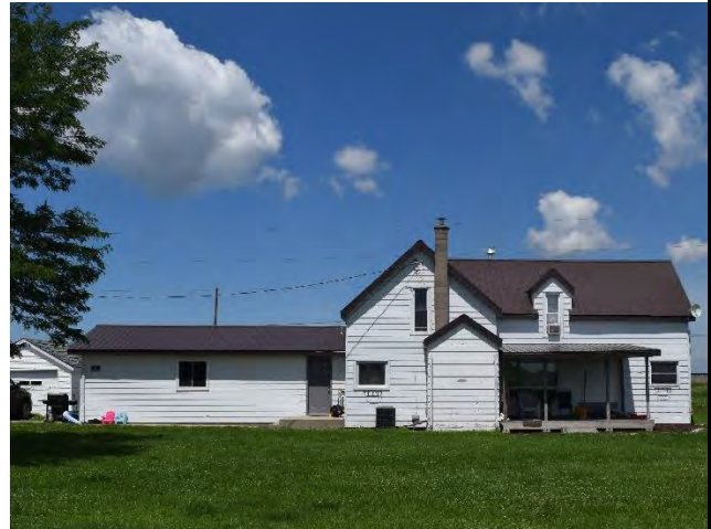
South (front) façade of house on property
