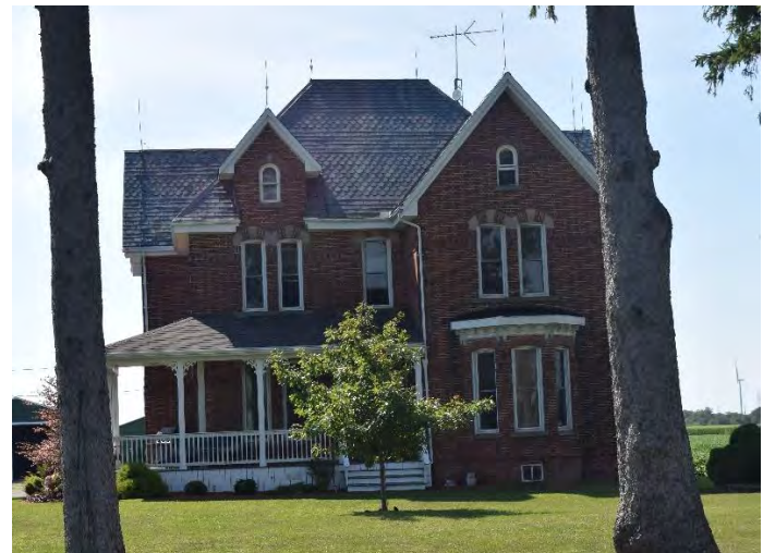
North (front) façade of house on property
