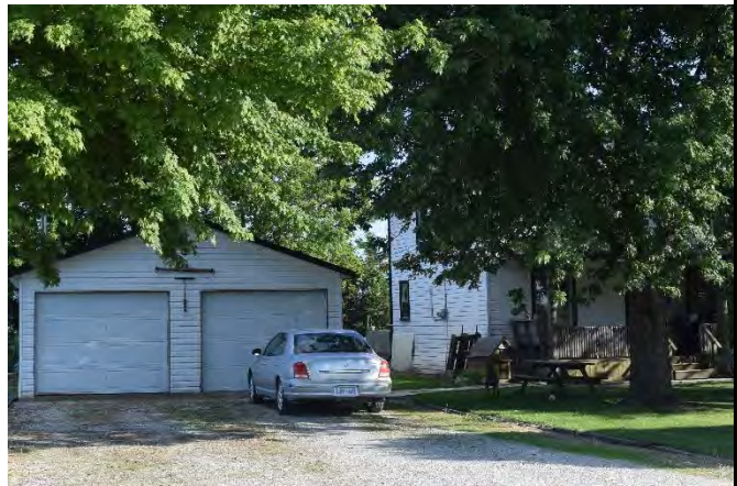
North (front) façade of house on property
