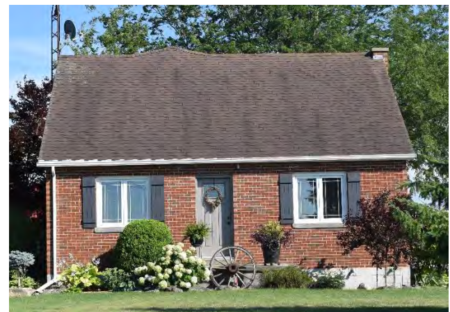
North (front) façade of house on property
