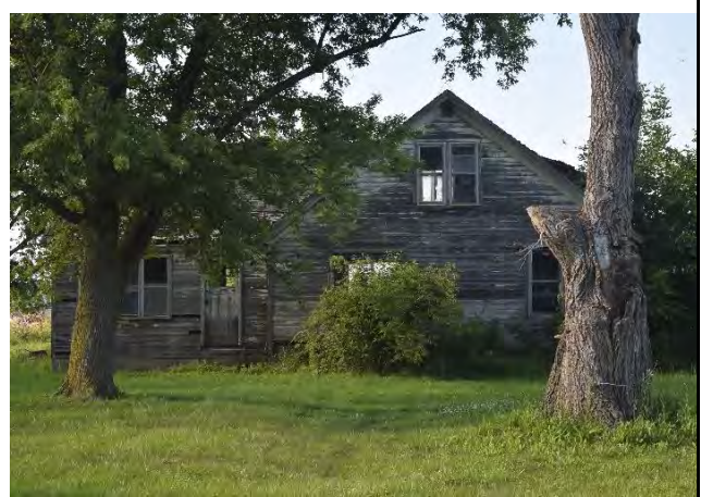
South (front) façade of house on property
