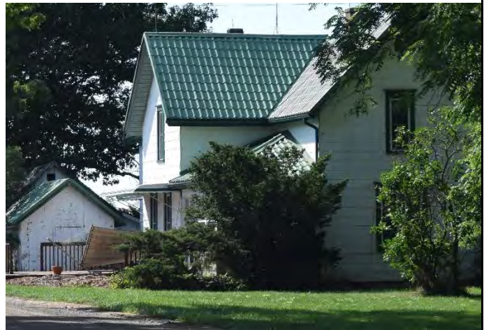
North (front) façade of house on property
