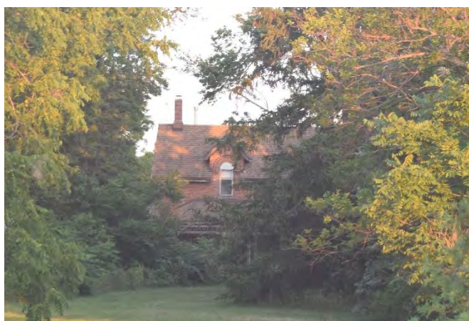
North (front) façade of house on property
