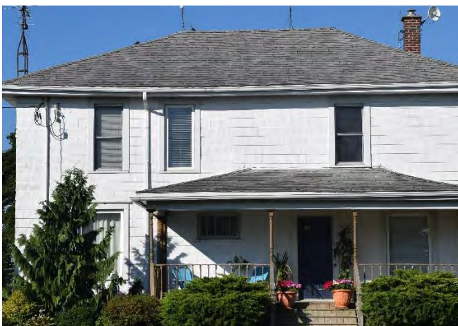
East (front) façade of house on property
