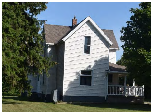
South (front) façade of house on property
