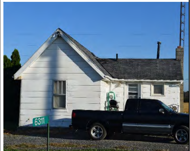
South (front) façade of house on property
