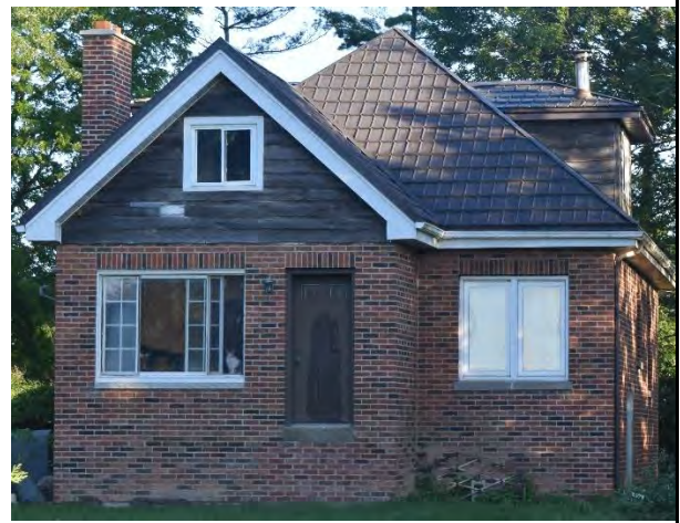
South (front) façade of house on property
