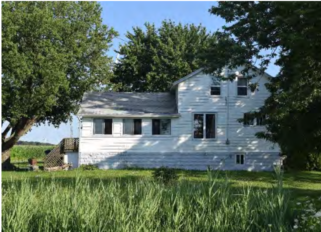
South (front) façade of house on property
