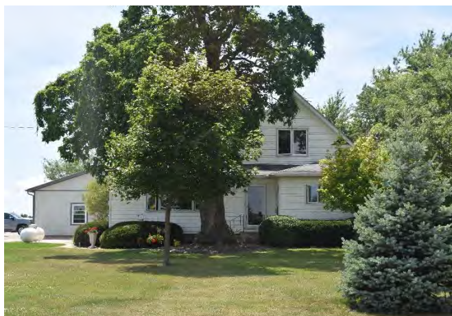
East (front) façade of house on property
