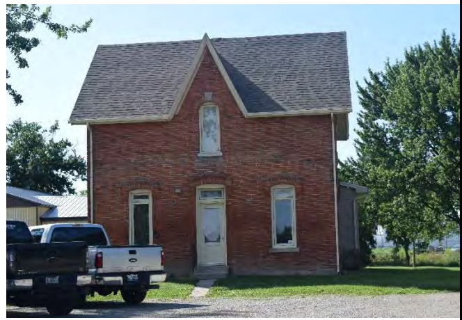
South (front) façade of house on property
