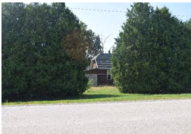
Associated structure on property, looking south from 8 Line
