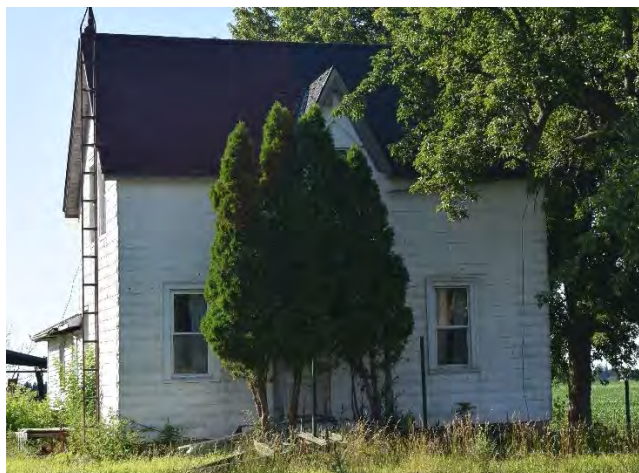
South (front) façade of house on property
