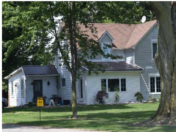
South (front) façade of house on property
