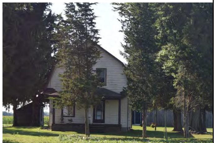
North (front) façade of house on property
