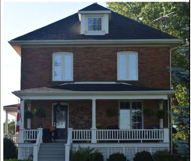
North (front) façade of house on property
