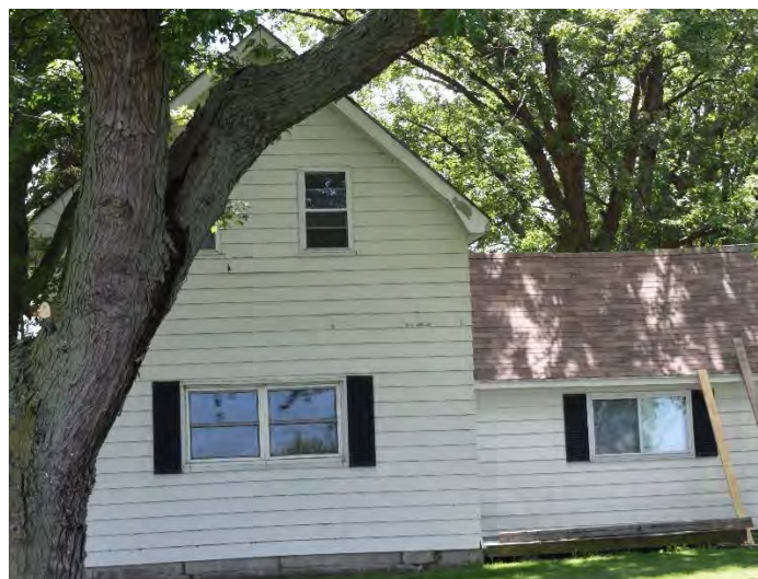
North (front) façade of house on property
