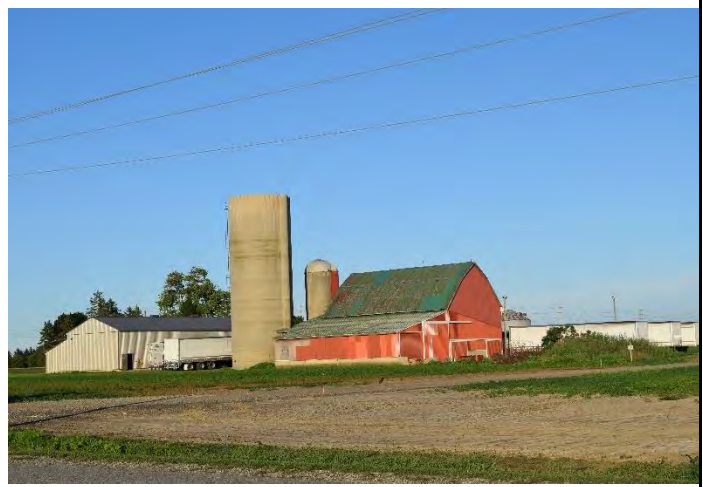
Associated barns on property, looking south from 5 Line East
