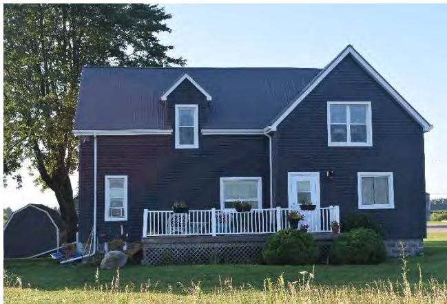
North (front) façade of house on property
