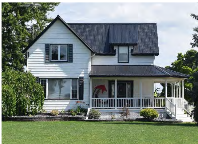
North (front) façade of house on property
