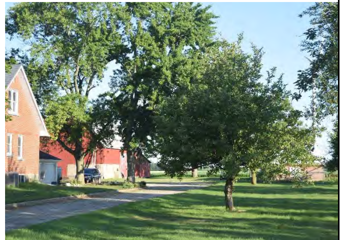
Associated barn on property, looking northwest from 7 Line West
