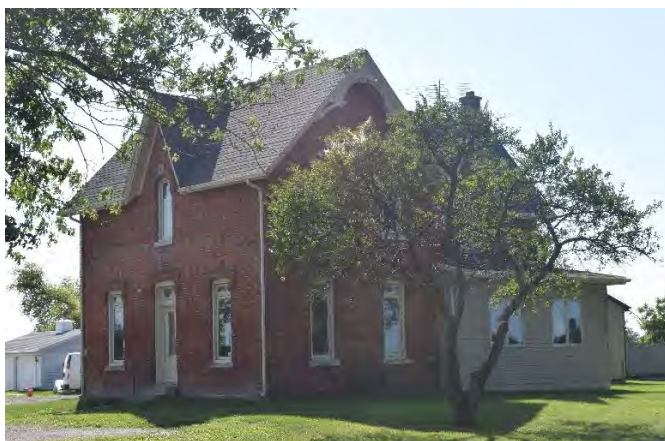
South (front) façade and east wall of house on property
