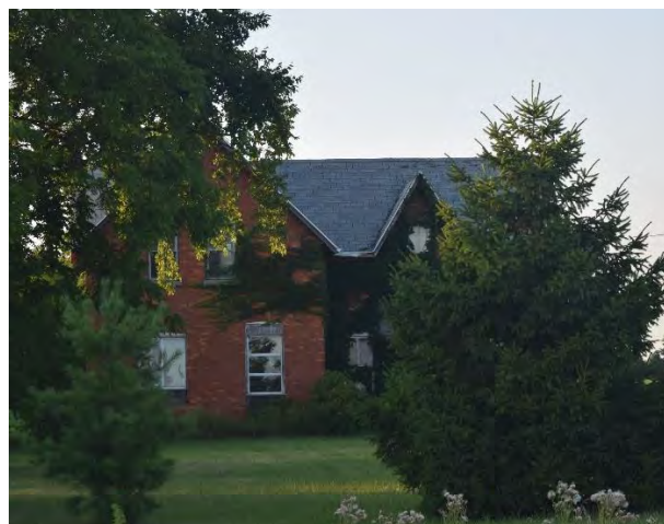
South (front) façade of house on property
