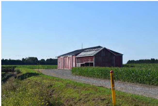
Associated barns on property, looking south from 9 Line
