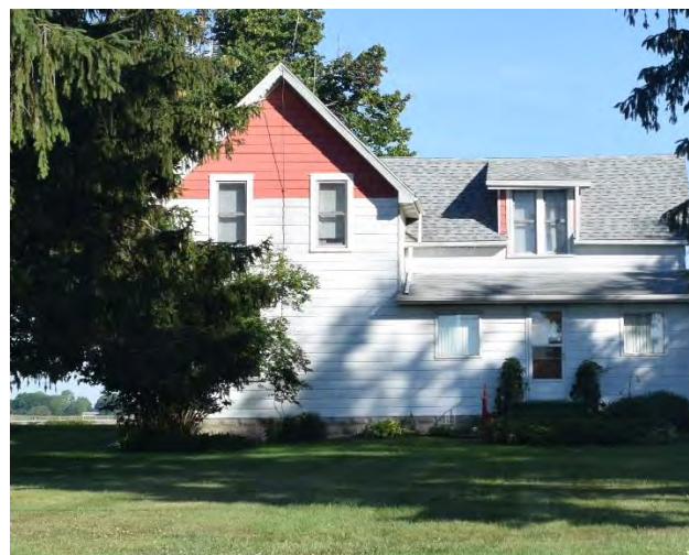
South (front) façade of house on property
