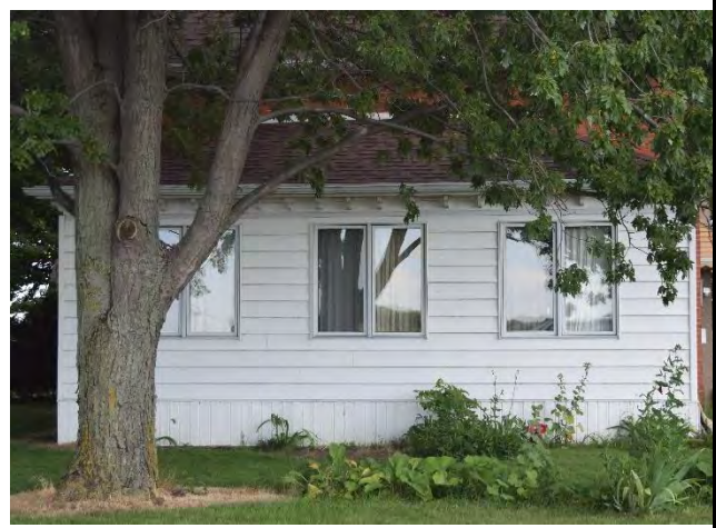
North (front) façade of house on property
