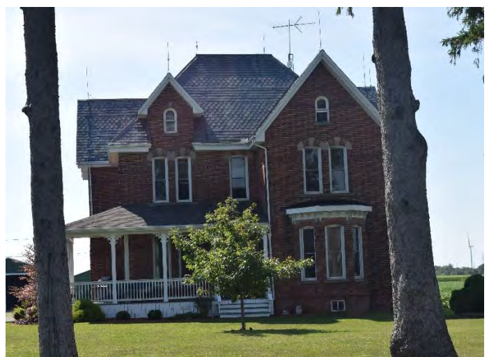
North (front) façade of house on property
