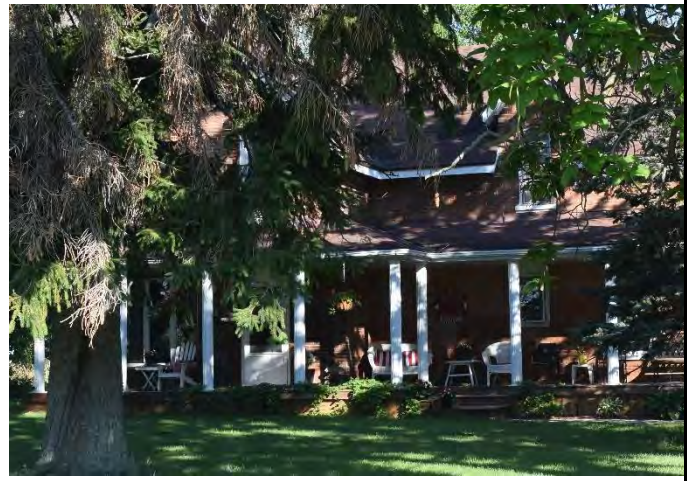
South (front) façade of house on property
