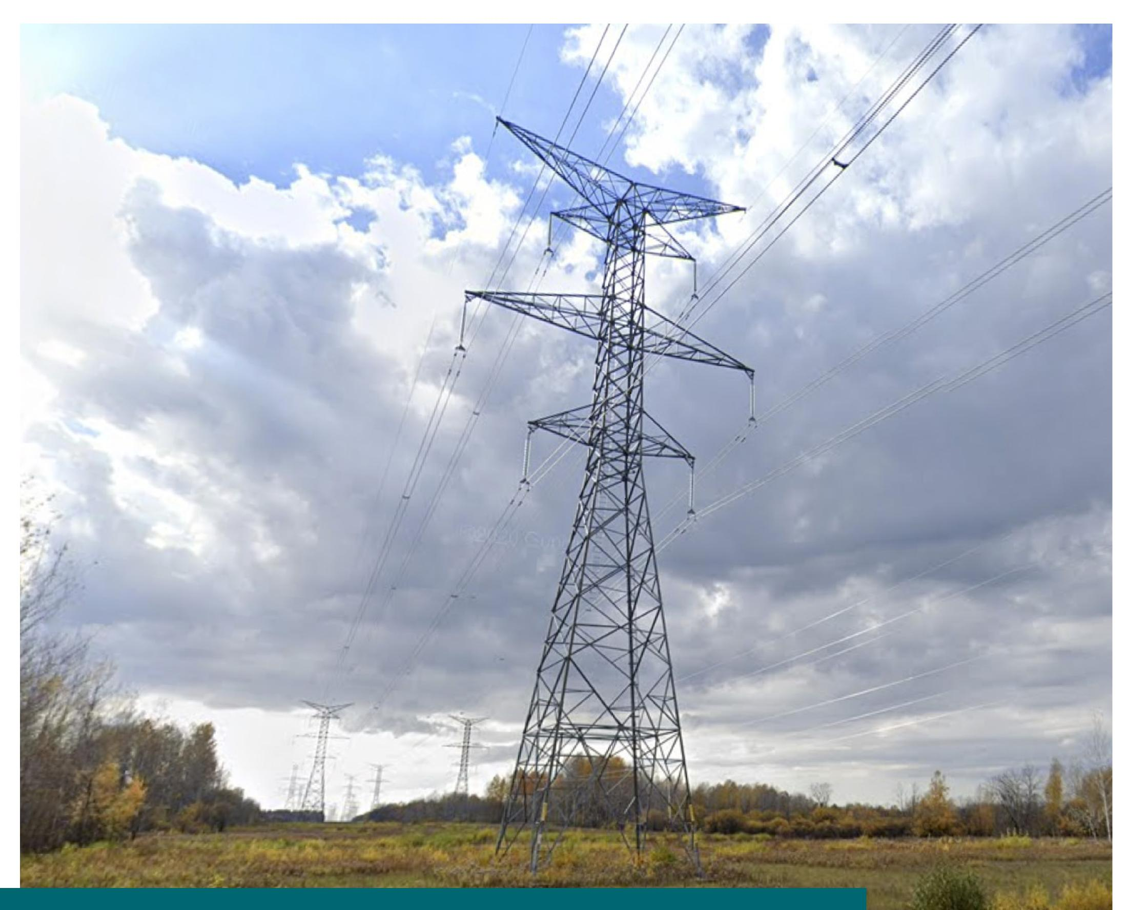
Example of twin bundled conductor on a transmission line between Hawthorne TS and the Quebec border
