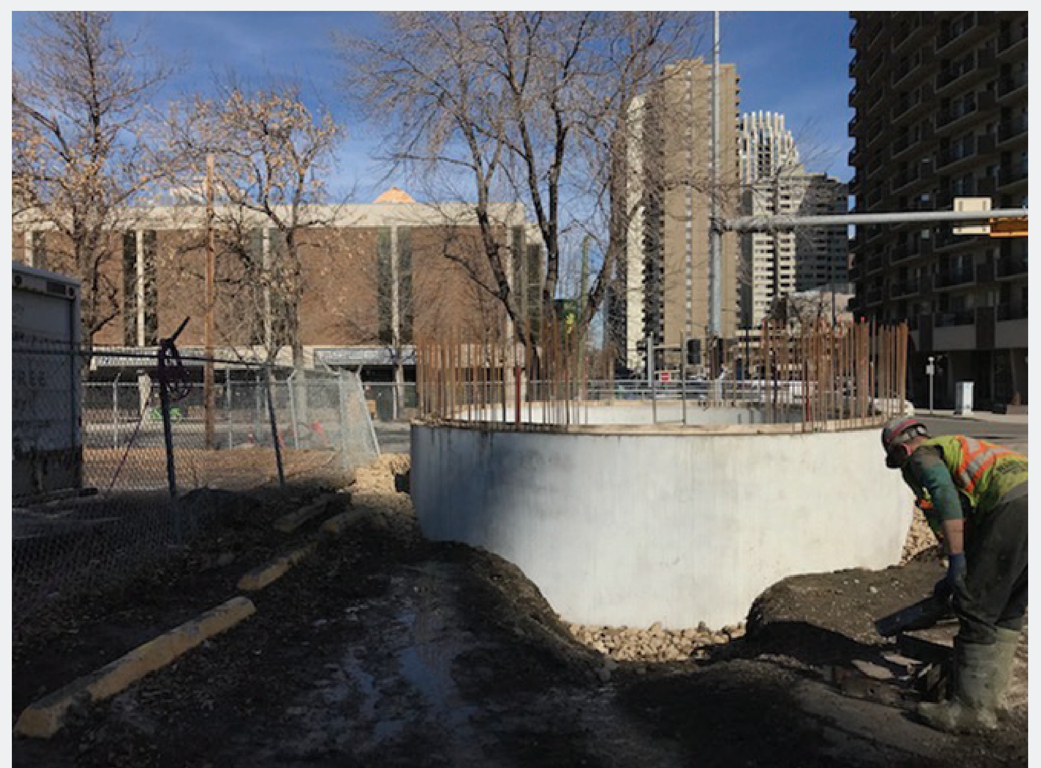
Example of shaft required for micro-tunneling construction
