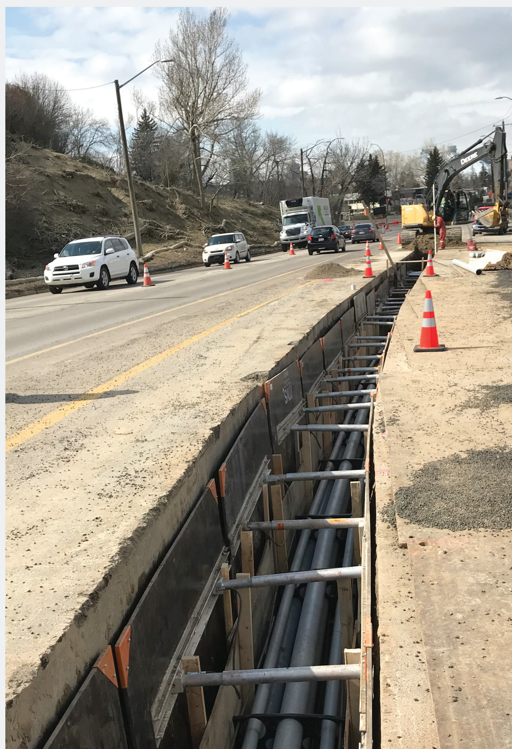
Example of open cut construction
