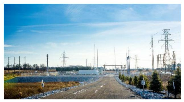
Figure 3: A Typical 230 kV Transformer Station
