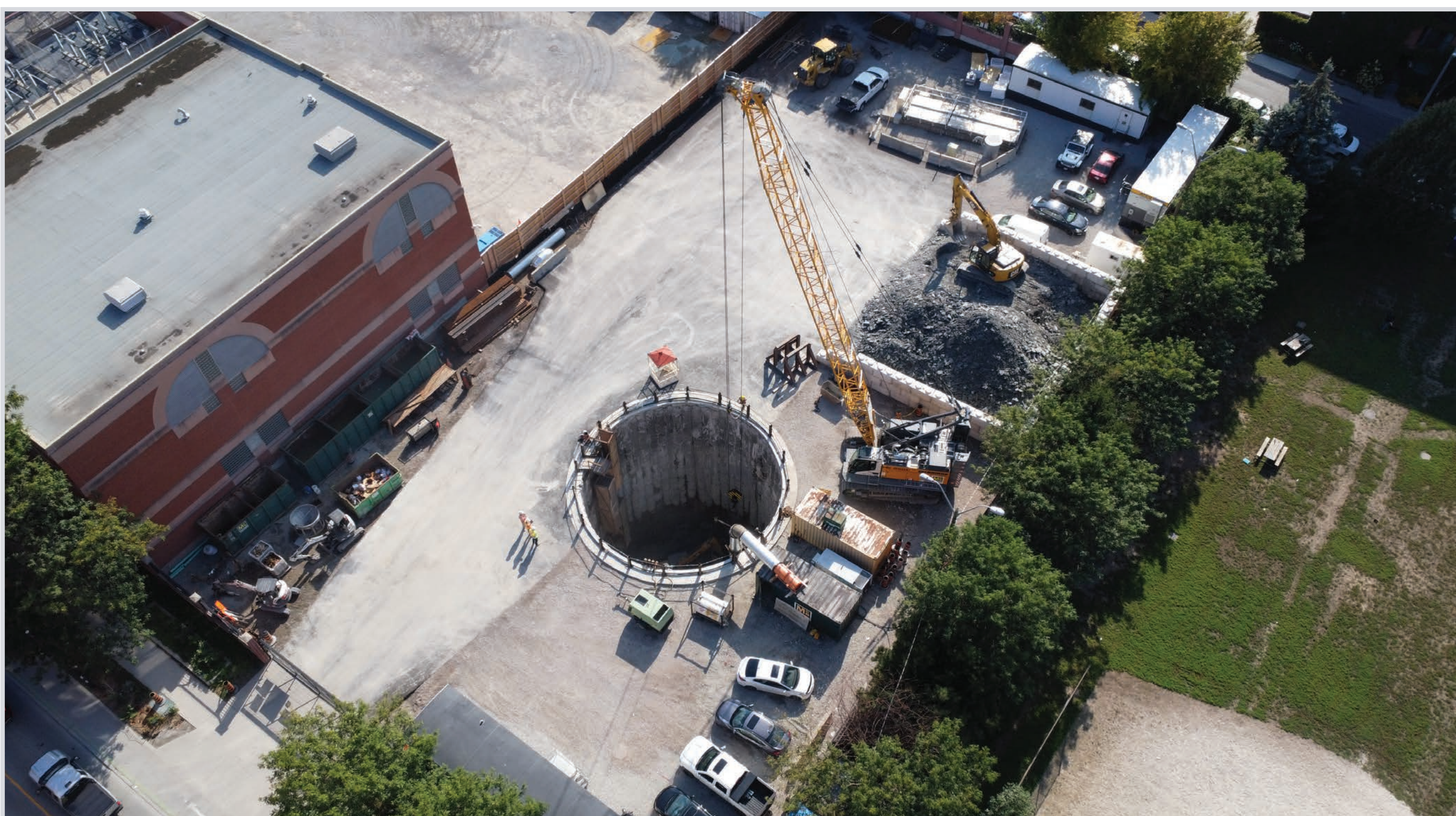
Example of a tunnel shaft during construction
