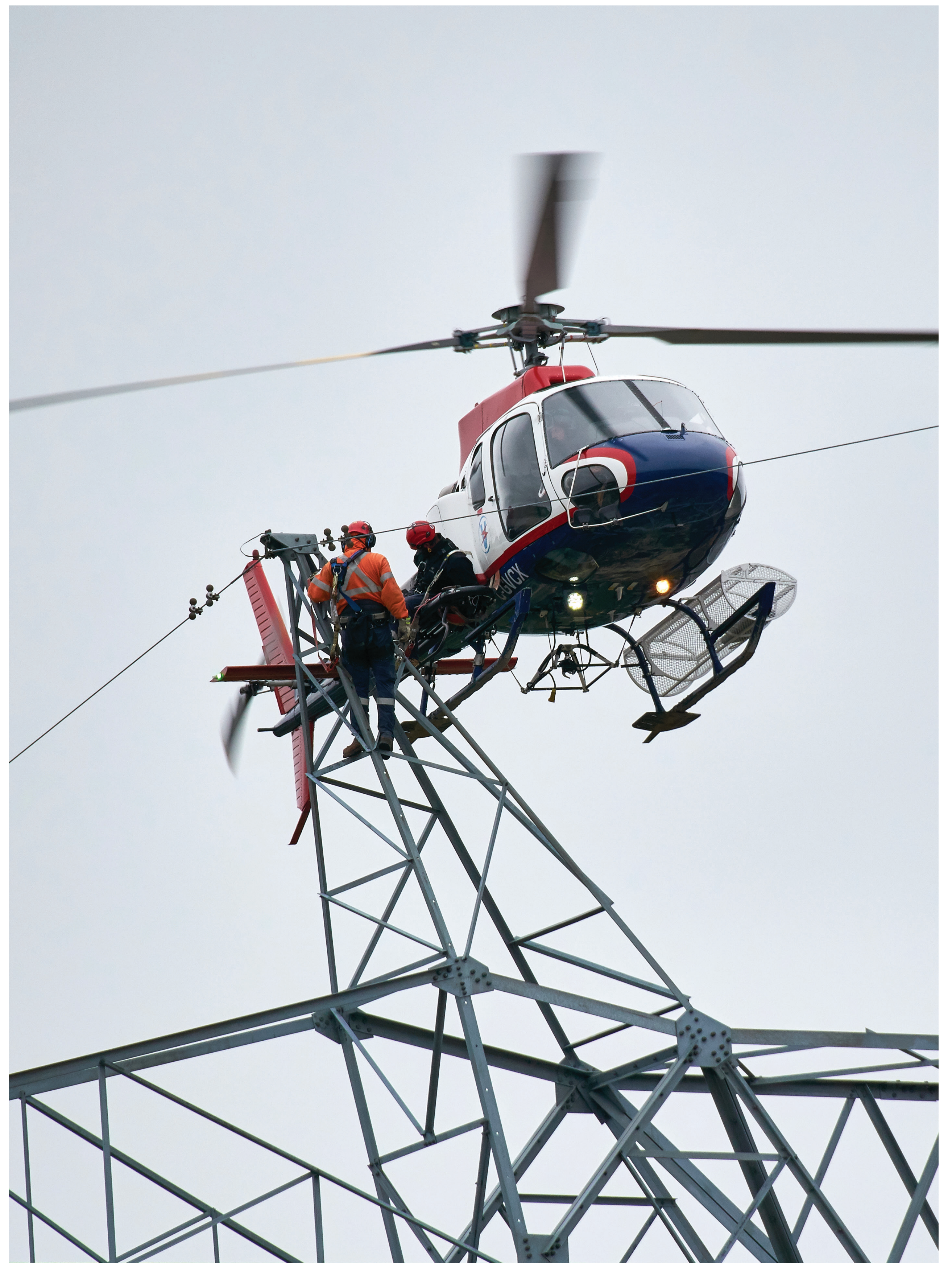
Helicopters are used to help string the line.
