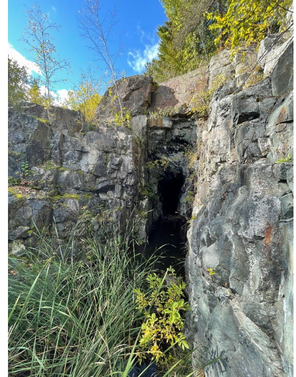
Photo 14: Spillway Inlet Activity Station Looking at Feature
