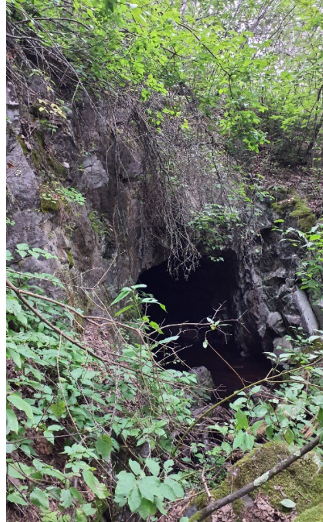
Photo 16: Spillway Outlet Activity Station Looking at Feature
