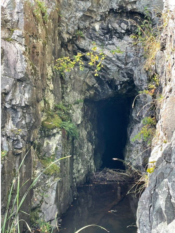
Photo 15: Spillway Inlet Activity Station Close Up of Feature
