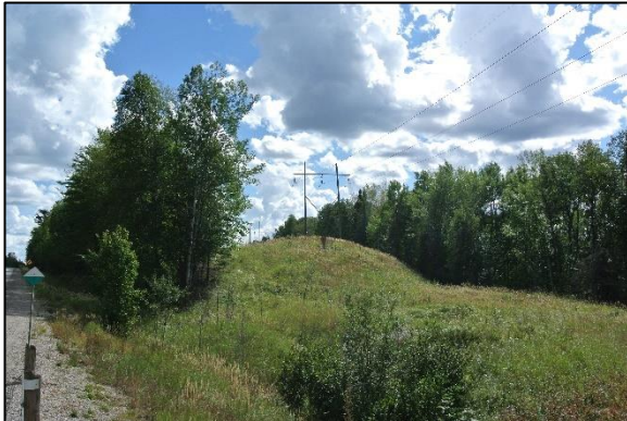
Photograph 11: View of existing transmission line corridor within Alternative Route 2B
