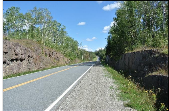
Photograph 10: Example of road within Alternative Route 2A
