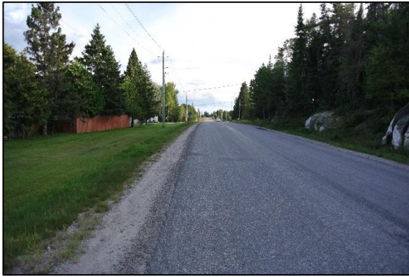
Photograph 15: Example of road within Alternative Routes 3A, 3B, and 3C
