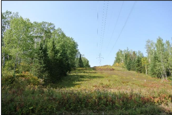
Photograph 1: View of existing transmission line corridor within Alternative Route 1
