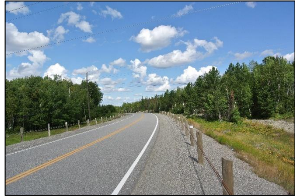
Photograph 14: Example of road within Alternative Route 2C
