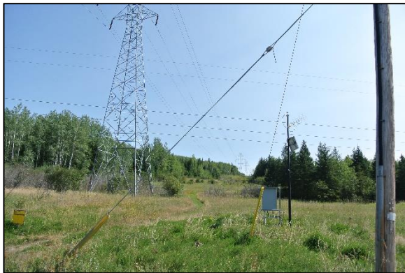
Photograph 3: View of existing transmission line corridor within Alternative Route 1A
