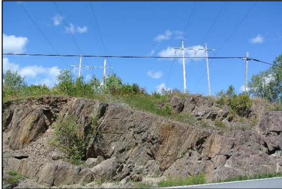
Photograph 9: View of existing transmission line corridor within Alternative Route 2A
