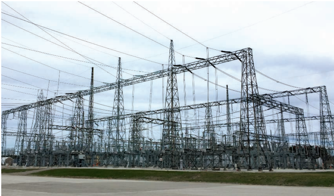
Current view inside Essa TS
