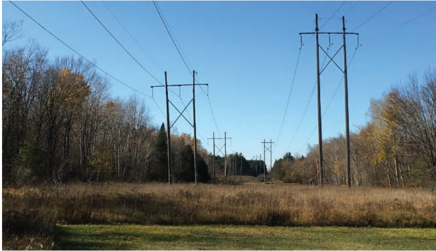
The existing structures are between 50-80 ft high
