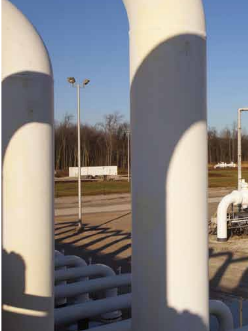
Natural gas storage facilities at Dawn, Ontario. Photo: Union Gas Limited
