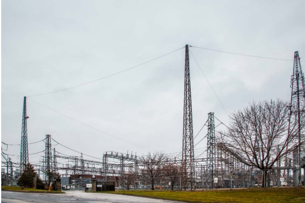
Figure 1-4: Photograph of Leaside TS
