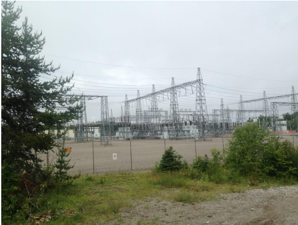
Photo 1: Existing Marathon TS, looking west from the entrance of Shack Lake access trail at Peninsula Road. July 9, 2017.
