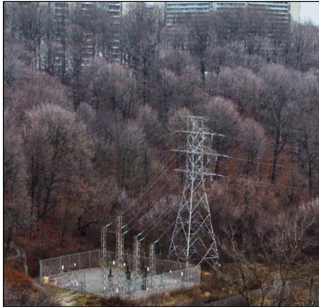
Figure 5-1: Photograph of Todmorden Junction in Toronto
