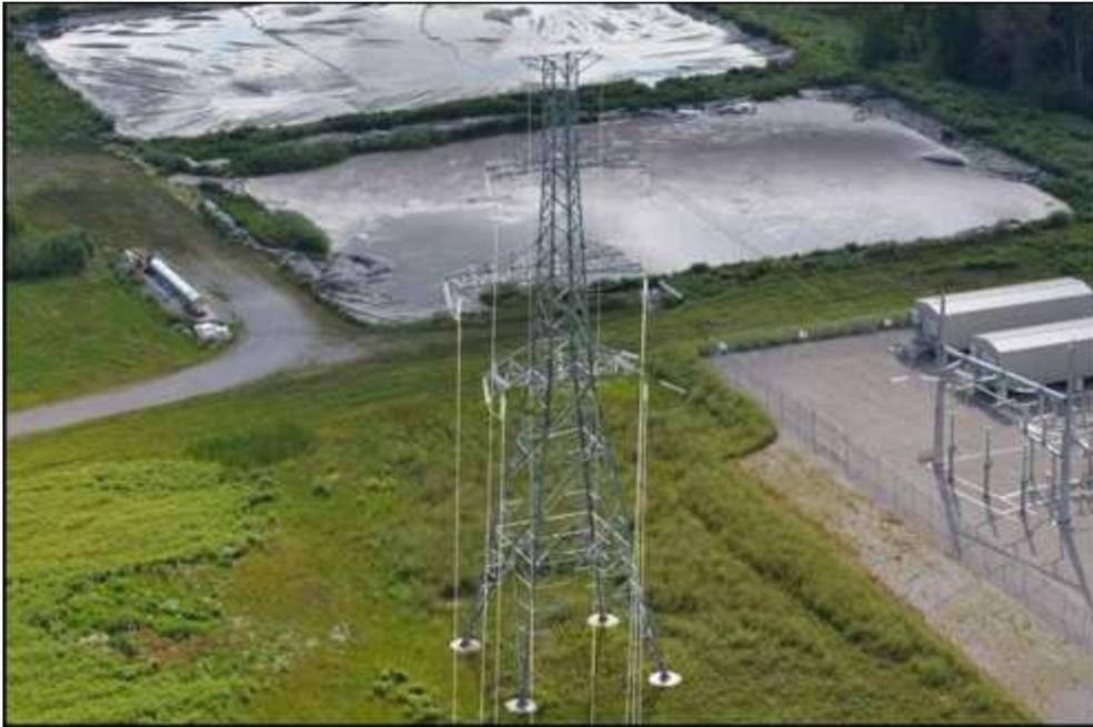
Figure 1-7: Example of a Typical Line Tap Structure
