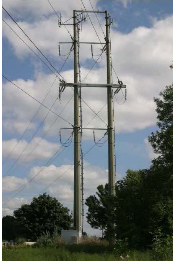
Figure 4-1: Photo of 230 kV Double Steel Pole Transmission Turning Structure
