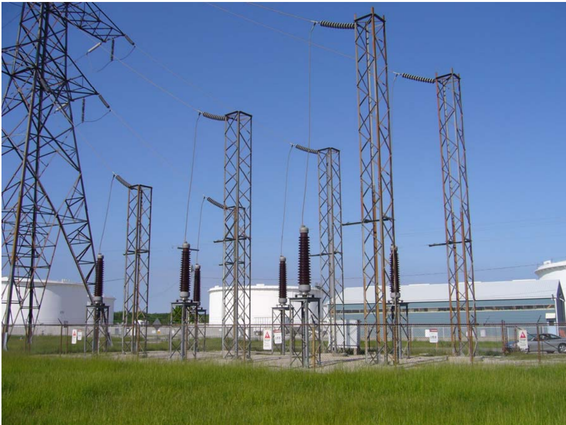
Figure 4-3: Photo of Cable Junction Converting 230 kV Overhead Line to Underground Cables
