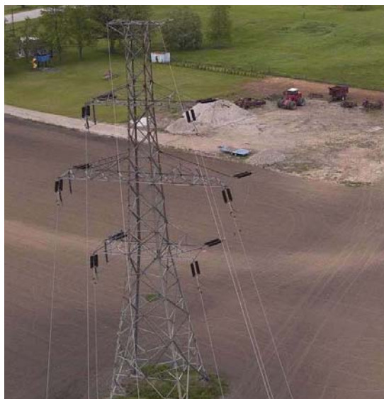
Figure 4-2: 230 kV Steel Lattice Anchor Tower
