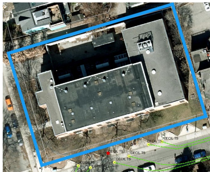
Figure 8-1: Cecil TS located in Downtown Toronto
