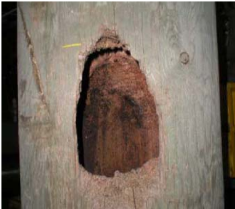
Figure 29: Woodpecker Damage
