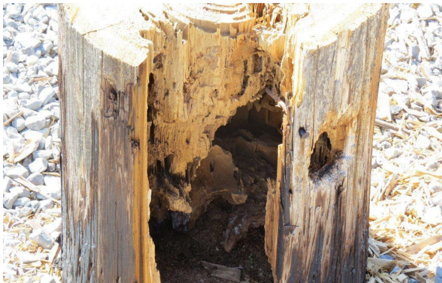
Figure 3: Stub From A Hollow MUS Structure That Was Replaced
