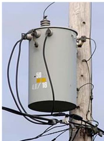
10 11 Figure 52: Picture of Pole-Top Line Transformer
