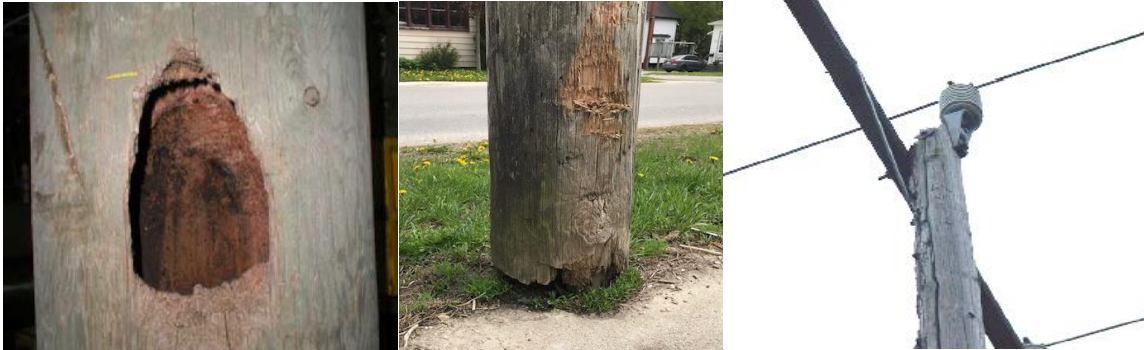
4 Figure 1: Examples of Poor-Condition Poles
