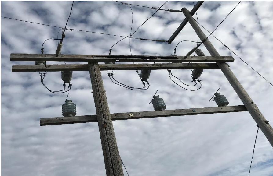
Figure 2: MUS Structure With Rotted Poles & Cross-Arms
