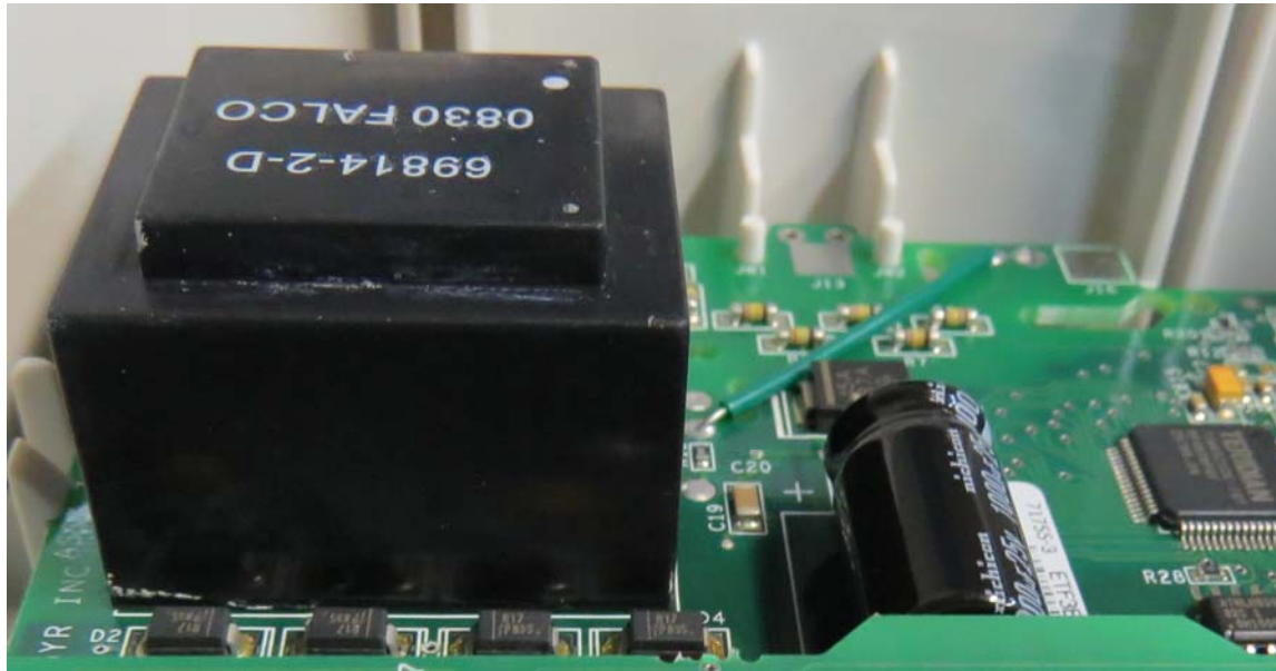
Figure 32. XFO failure on meter #19 – 2970501
