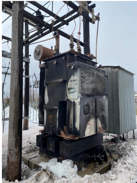
Figure 2: Failed Schreiber Winnipeg DS R1 Regulator (2020)
