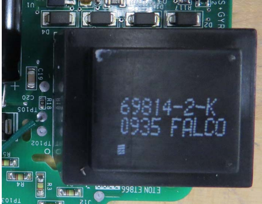
Figure 2. Transformer with primary winding open
