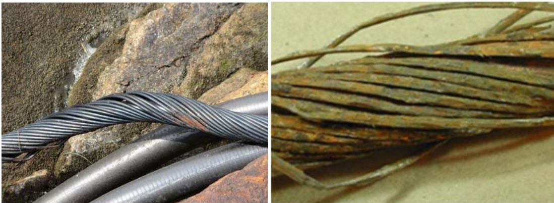
7 Figure 42: Example of (Left) an Exposed Cable Showing Initial Signs of Corrosion, and (Right) a 8 Corroded Cable with Significant Damage
