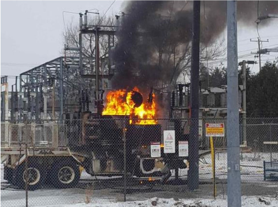
Figure 4: MUS 26 Transformer Failure
