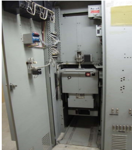
Figure 7: Picture of a Metalclad Breaker
