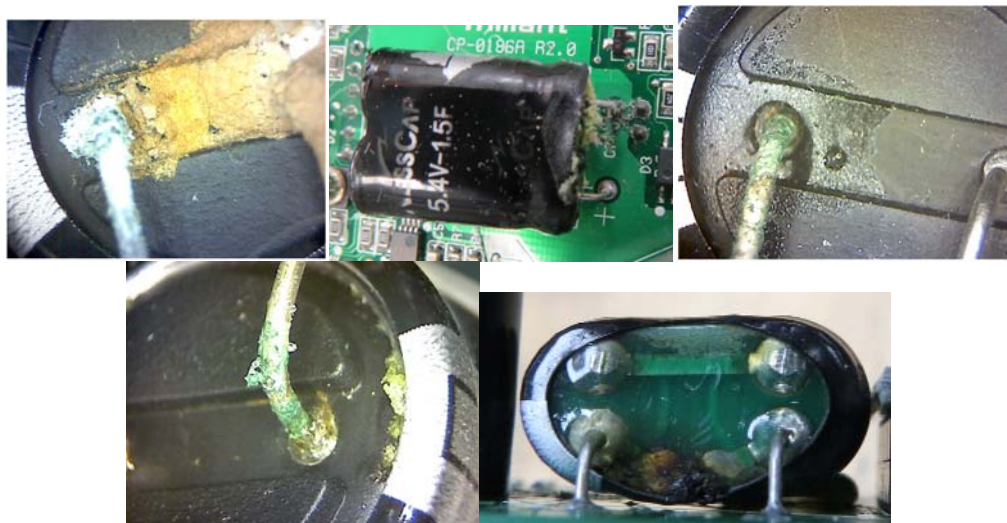
Figure 8. Capacitor failures in GEN1 meters
