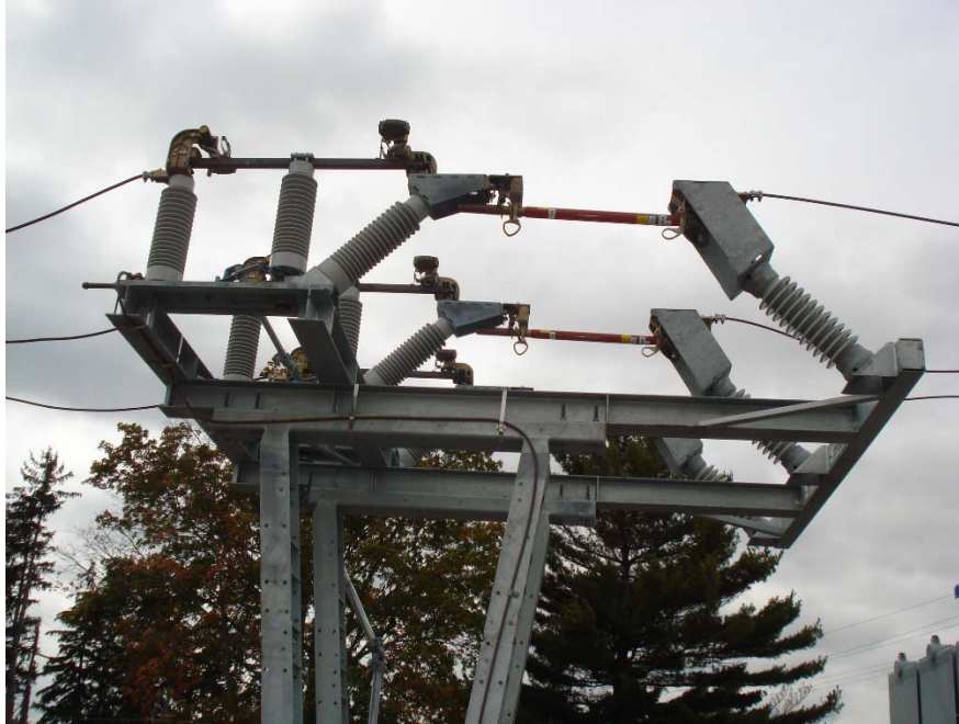
Figure 12: Picture of Station Switch and Fuse Combination
