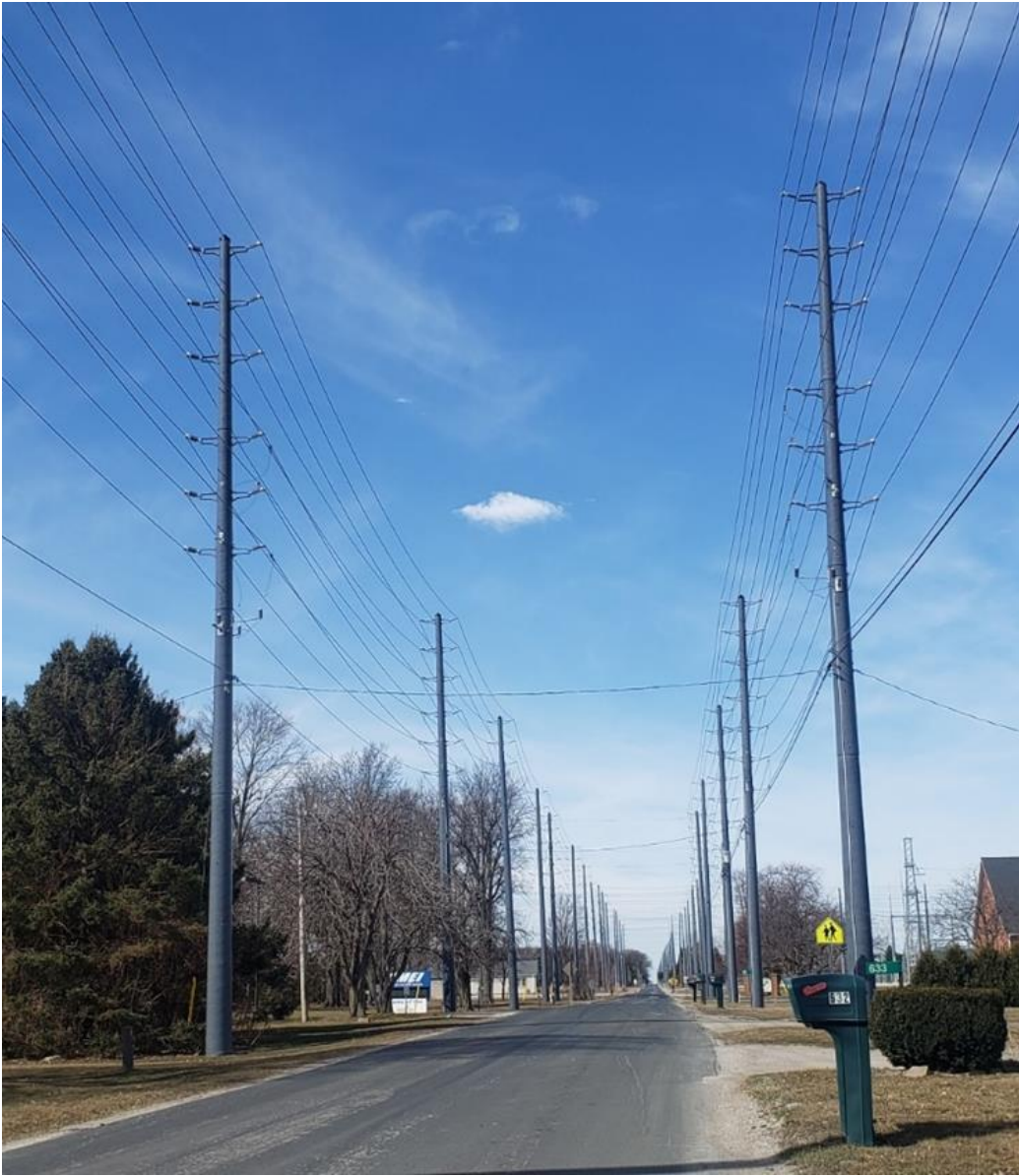
Figure 5: Leamington TS #1 Overhead Circuit Congestion
