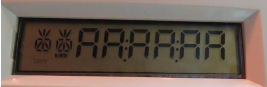
Figure 25. Missing segments on meter J2573239
