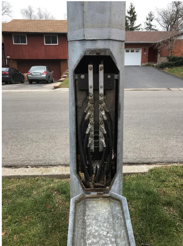
5 Figure 2: Pole Transformer
