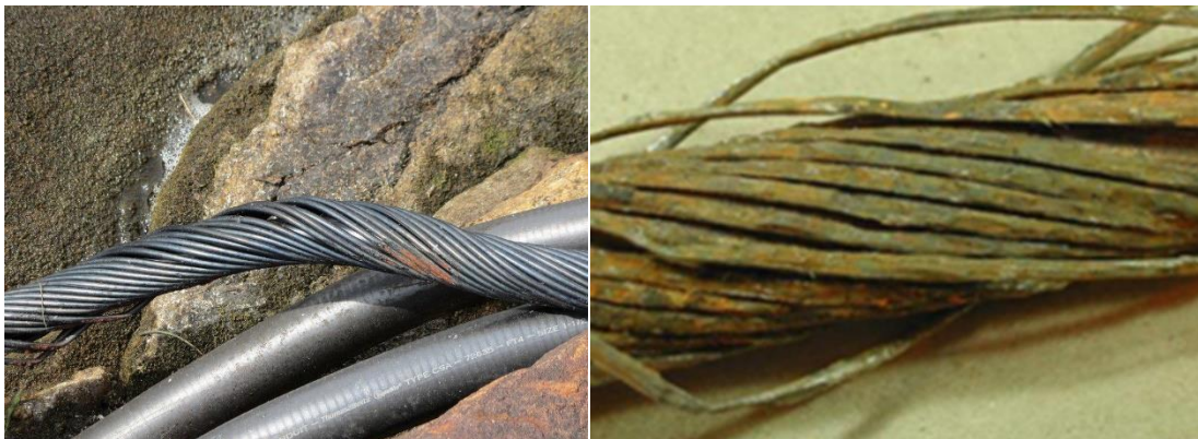
19 Figure 1: Example of (left) an Exposed Cable Showing Initial Signs of Corrosion, and (Right) a 20 Corroded Cable with Significant Damage
