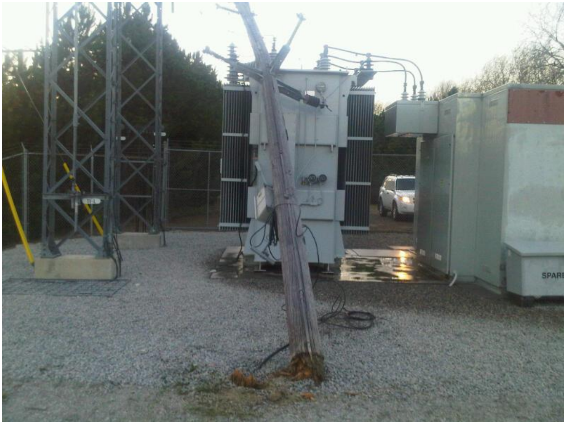
Figure 4: Broken MUS Pole at Bolton King DS
