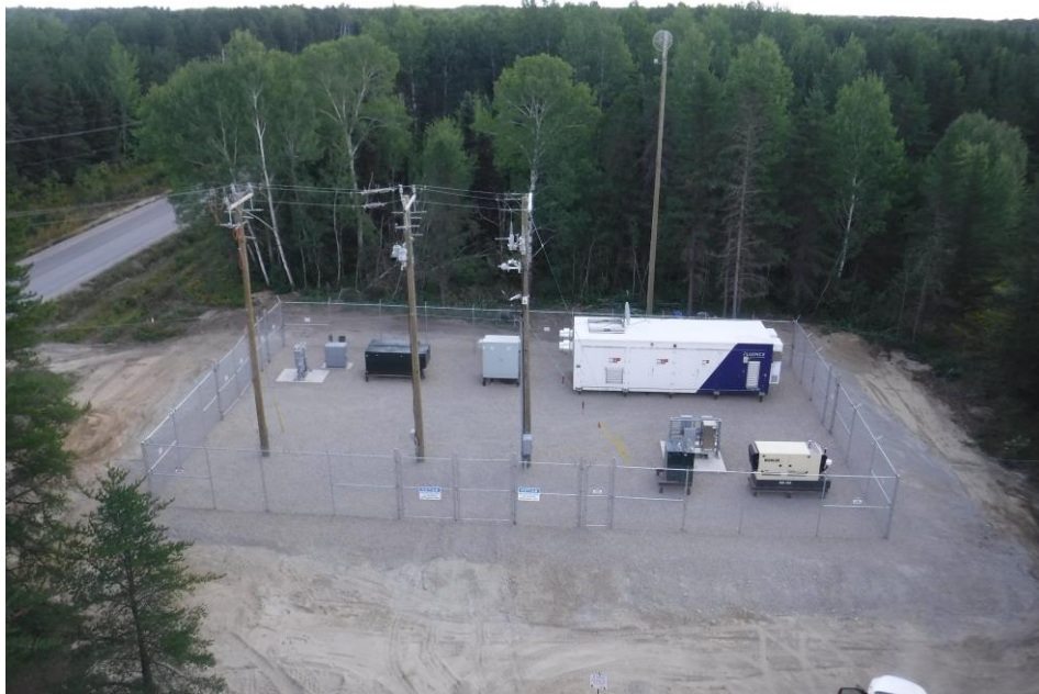
Figure 1: Aroland Battery Energy Storage System
