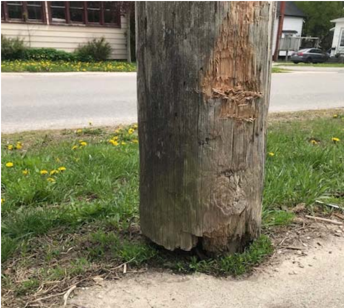
Figure 30: Ground Line Surface Rot
