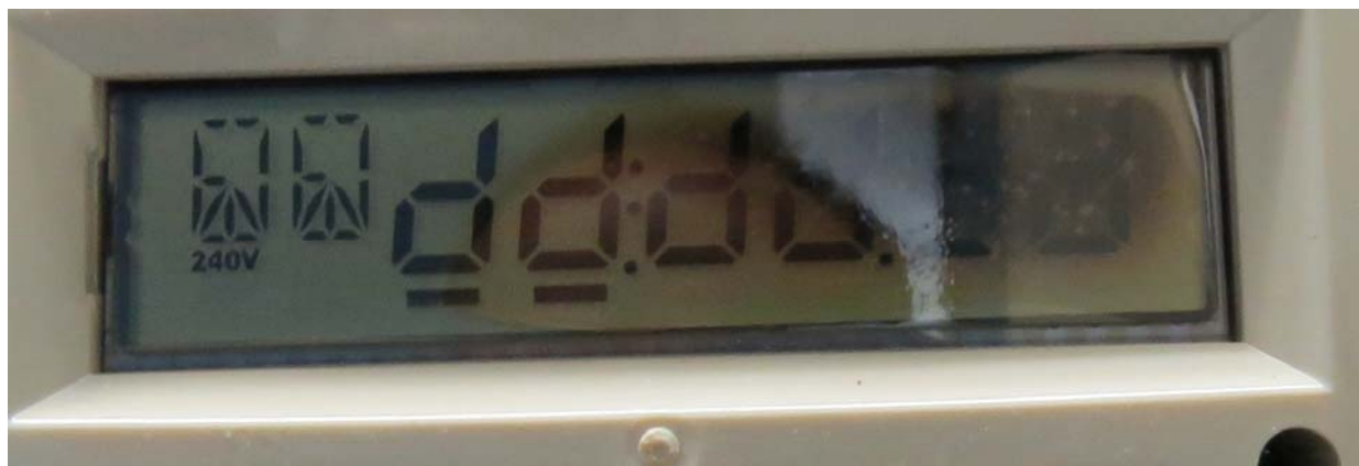
Figure 48. Meter J2965870 with missing segments
