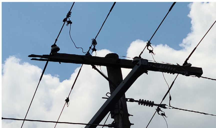
Figure 38 – Cross Arm in Poor Condition
