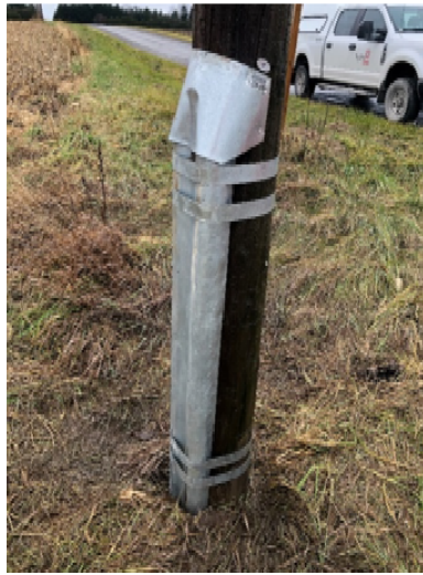
Figure 36: Mechanically Refurbished Pole
