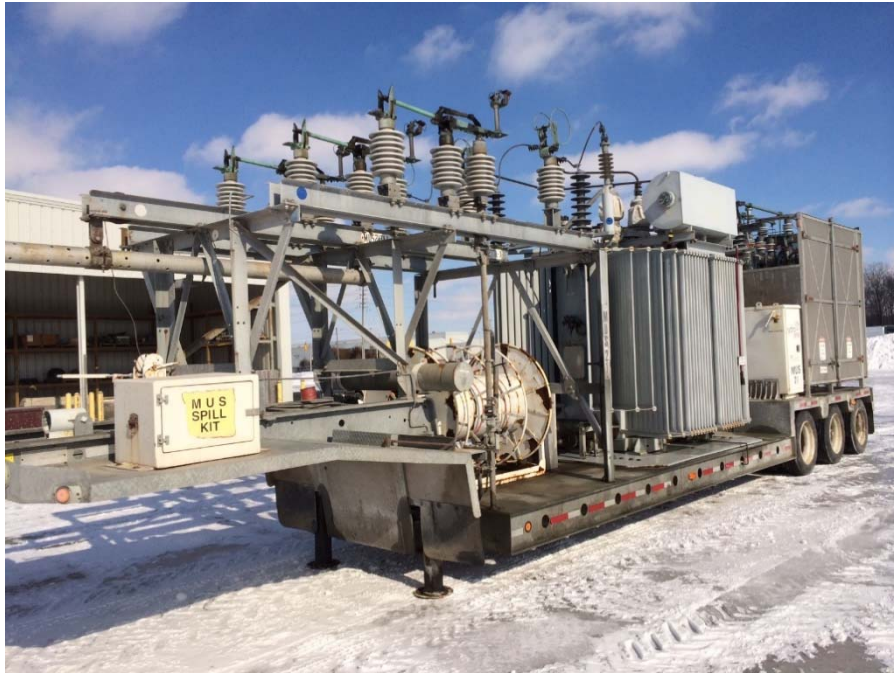
Figure 16: Picture of Mobile Unit Substation
