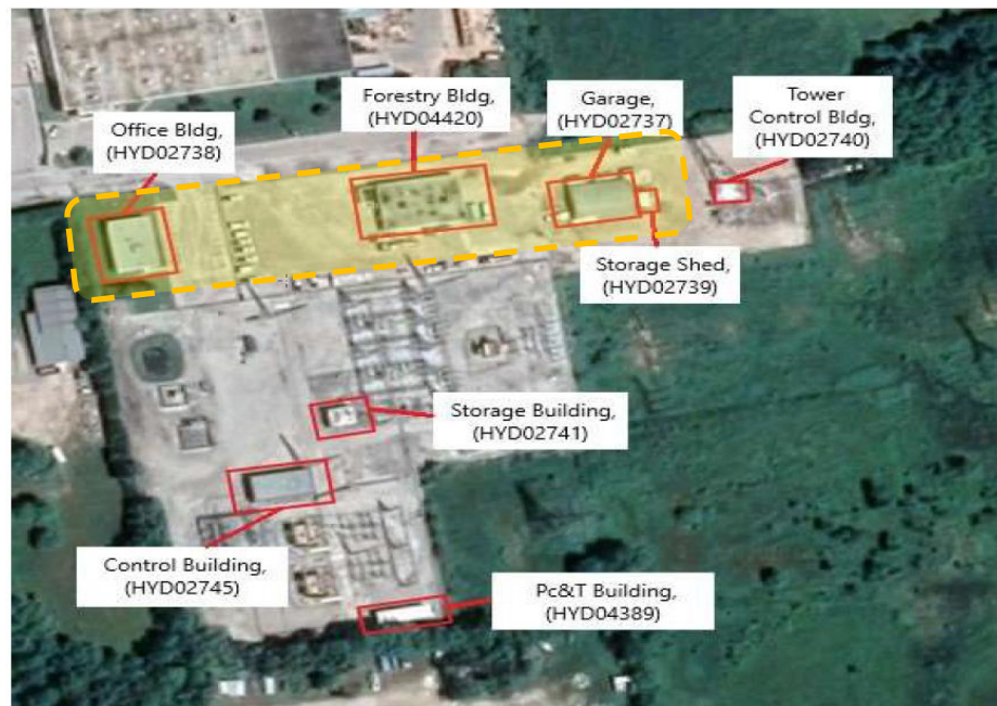
4 Figure 7: Aerial View of Owen Sound TS; Highlighted Area Indicates Buildings that are 5 Expected to be Decommissioned as Part of the Consolidation
