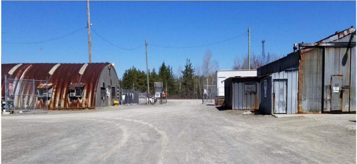
3 Figure 4: Ground View of Current Hanmer Work Centre Showing from the Left: Quonset Hut, 4 Washroom (White) Trailer and Condemned Building on the Right
