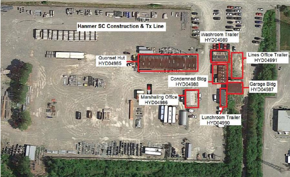
1 Figure 3: Aerial View of the Hanmer SC Construction and Transmission Lines Site.
