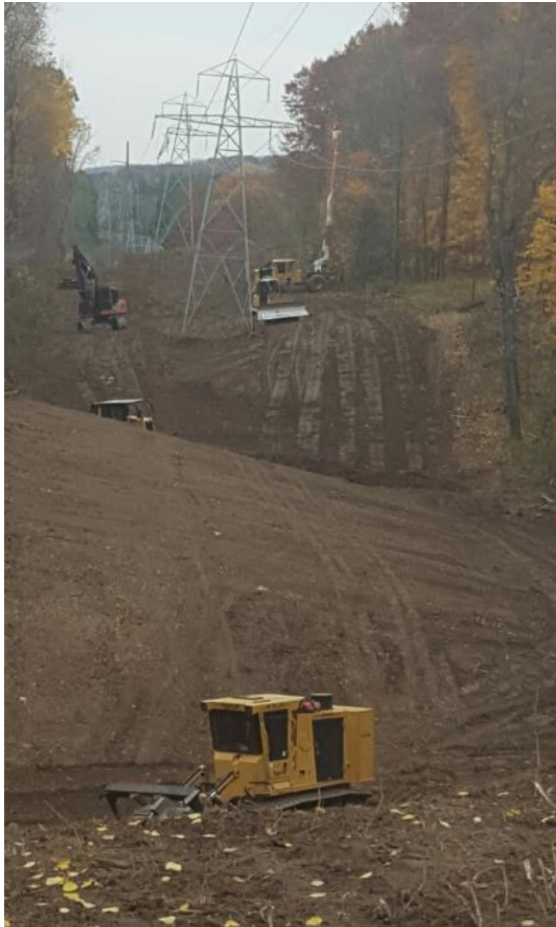
Example of transmission ROW work
