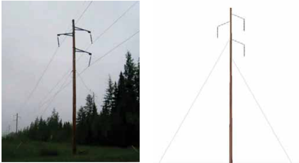
7 Figure 1: Picture of a single-pole suspension structure along the H9K circuit with steel 8 harp arms adjacent to a virtual rendition of the same structure.
