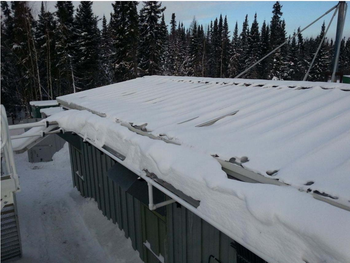
Photo#17 – Exposed Fuel Line Tray & Visible Heat Loss (Weagamow)
