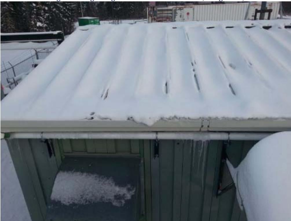
**Figure 10: Exposed Fuel Line Tray & Visible Heat Loss (Weagamow)**
