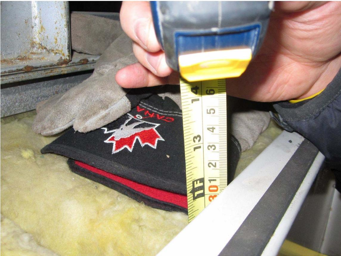
Photo#2 – Existing Roof Insulation Thickness (Kingfisher Lake)
