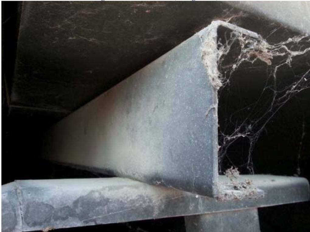
**Figure 8: Insufficient Air Space (Weagamow)**
