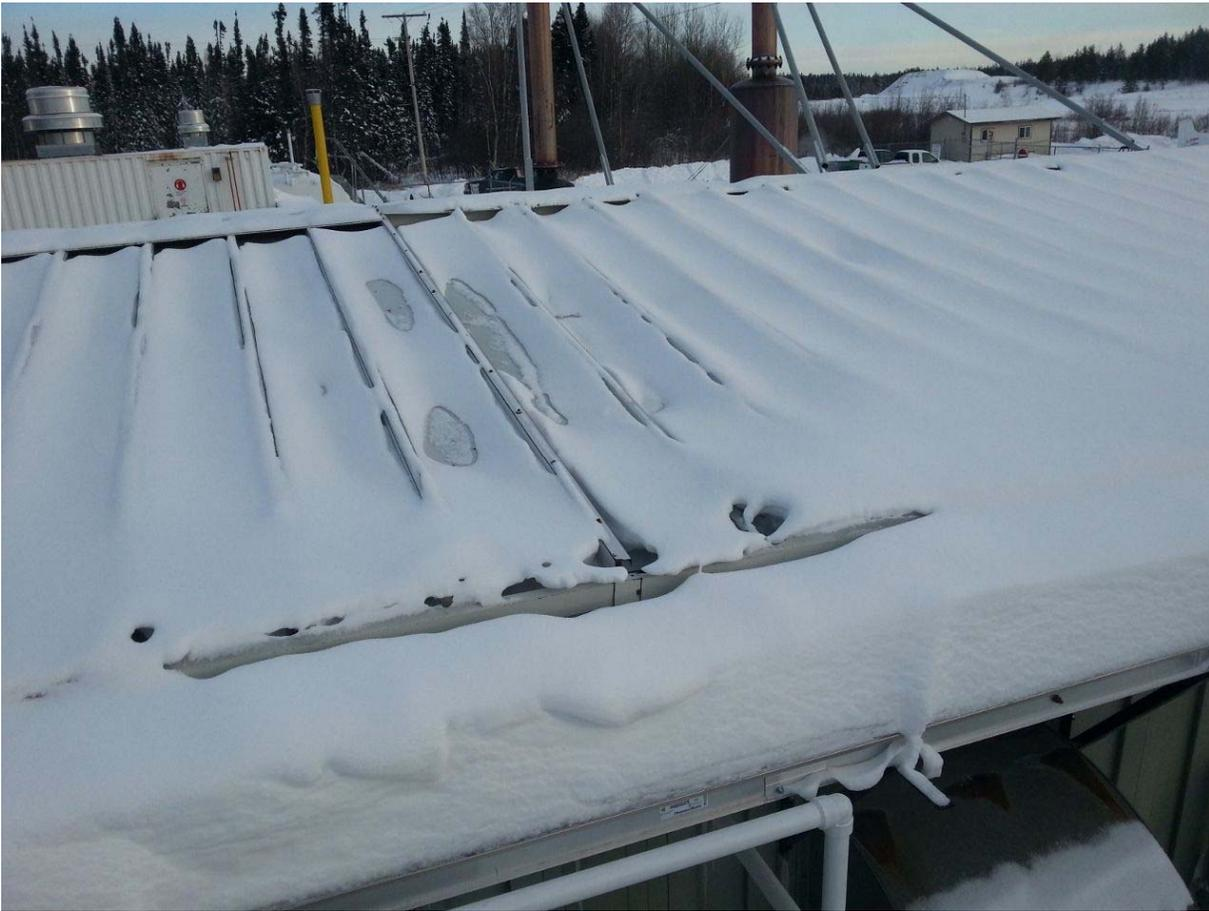
Photo#18 – Visible Heat Loss & Roof Panel Deterioration Signs (Weagamow)
