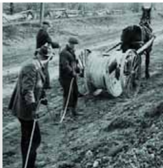
Left: Using single-horse power, these men made good progress in laying cable near Beamsville, Ontario, on November 22, 1923.
