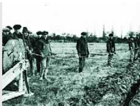
Left: December 7, 1921. An early method of spooling out cable.
