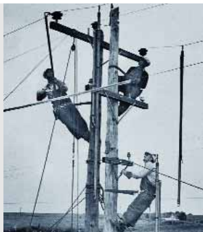
Left: Ontario Hydro linemen up the pole on June 11, 1947, were using hot line tools to work on "live" lines.
