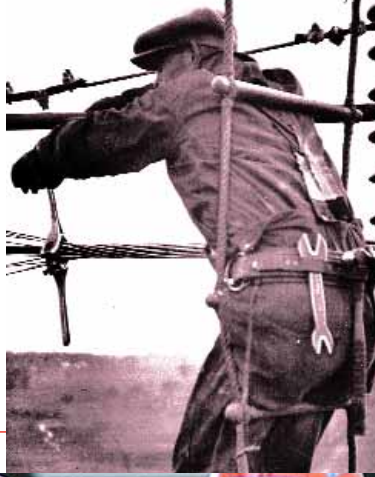
Left: This lineman was twisting absorber rods on cables when this picture was taken on January 18, 1932.
