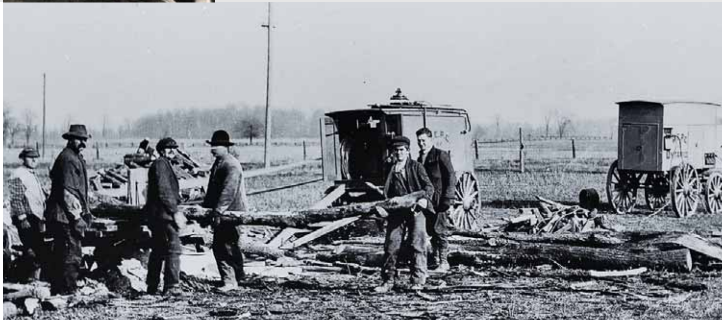
Above: Two units of the Adam Beck "Circus," which carried various appliances to the farms of Ontario to provide on-the-spot demonstrations, can be seen in the background of this photo taken in 1912. When they saw how easy it was to saw wood with Hydro, fewer and fewer farmers had axes to grind.
