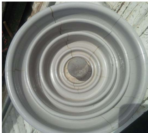
20 21 Figure 40: Porcelain Insulator Unit Affected by Cement Expansion
