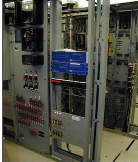
Figure 13C: Microprocessor Based Protection Scheme
