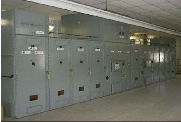
Figure 6C: Metalclad Circuit Breakers
