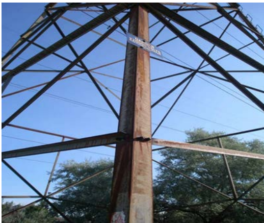
Figure 31C: Steel Tower with Corrosion
