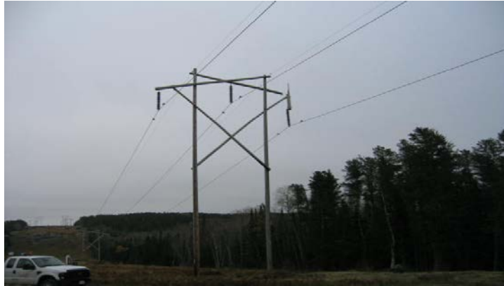
Figure 25C: 230 kV Gulfport Structure (with defective/failed cross-arm)
