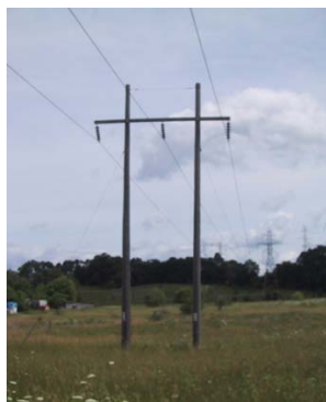
Figure 25A: Wood Pole H-Frame Structure
