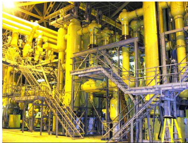
Figure 6E: 500kV GIS Circuit Breakers
