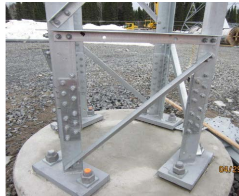
Figure 31B: Hot Dip Galvanized Steel Tower Structure
