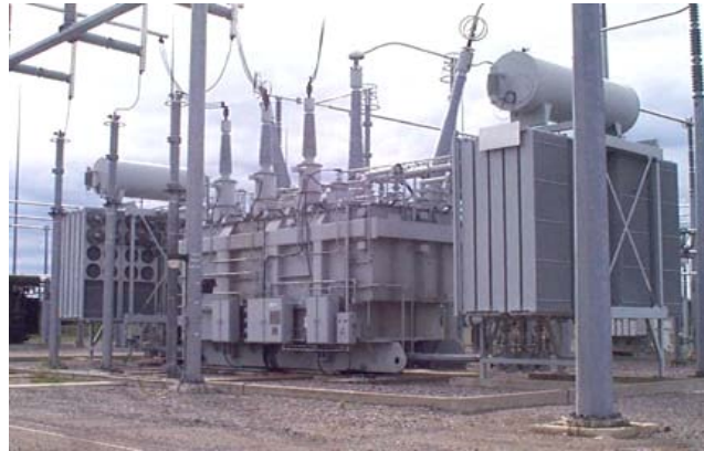
Figure 1: 500/230 kV Autotransformer
