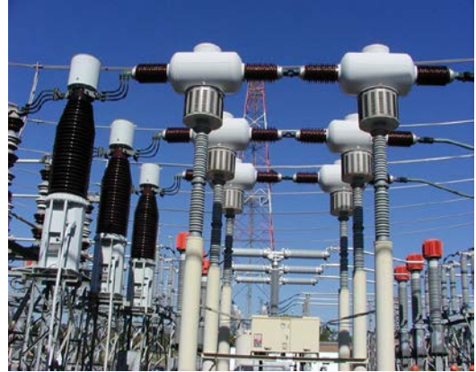
Figure 6D: Air Blast Circuit Breakers
