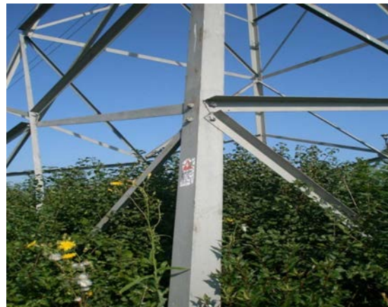
Figure 31D: Steel Tower Recoated
