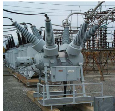
Figure 6B: SF6 Circuit Breaker
