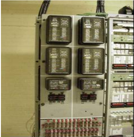
Figure 13A: Electromechanical Relay Panel
