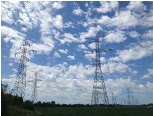
Figure 31A: Steel Tower Structure
