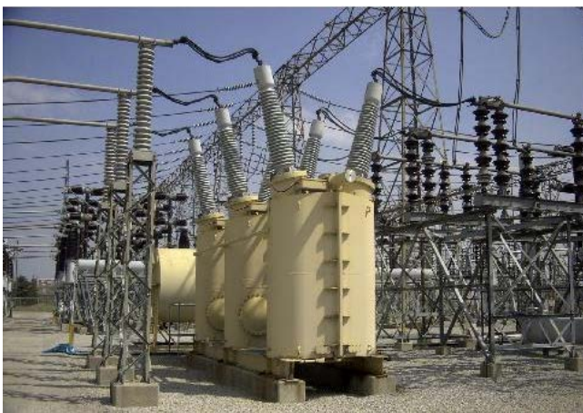
Figure 6A: Oil Circuit Breaker
