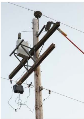
Figure 8 - Monitoring voltage distortion at feeder capacitor installation. Excessive level of harmonics may damage capacitors and negatively affect the feeder supply voltage profile.
