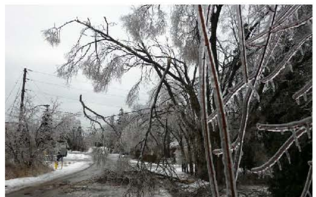
Figure 4 - Electrical distribution feeder damaged by ice-storm. Even regular tree trimming programs cannot always prevent power outages.
