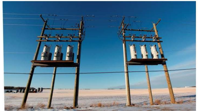
Figure 10 - In-line voltage regulators used by power utilities to improve voltage profiles on long distribution feeders
