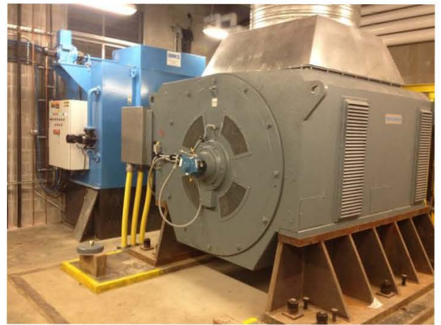
Figure 5 - Large 5000HP electric motor. Start, stop or cyclical loading of such motors may cause noticeable short duration sags in supply feeder voltage
