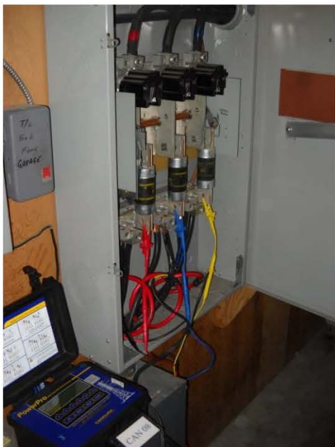
Figure 9 - Monitoring power quality at customer electrical installation
