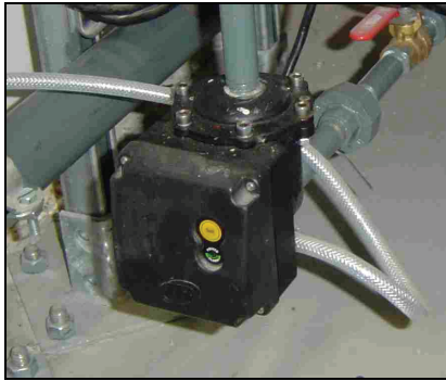
Figure 14 - Example of Zero Air Loss Drain
