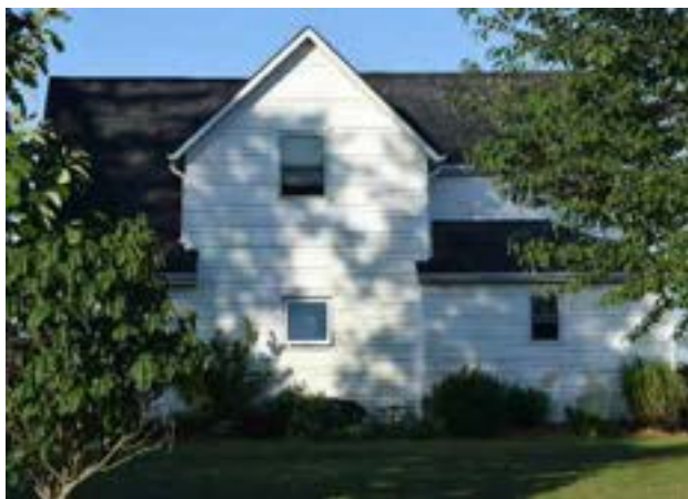
East (front) façade of house on property
