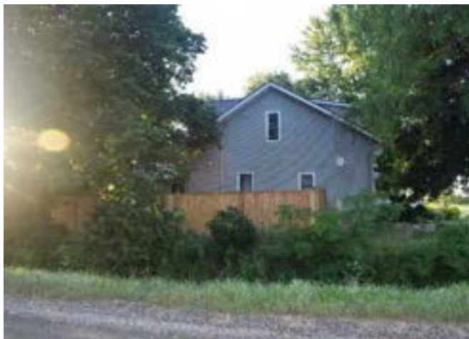
North wall of house on property
