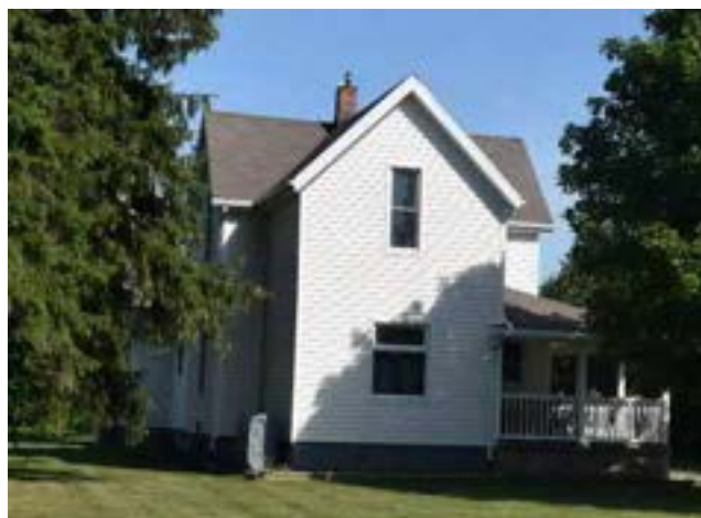
South (front) façade of house on property
