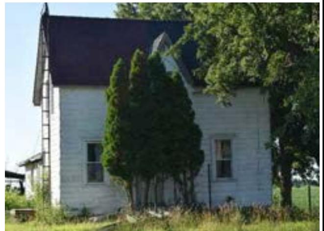
South (front) façade of house on property
