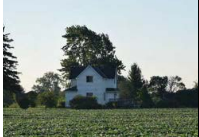
North façade of house on property
