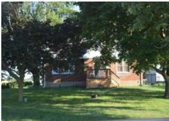
South (front) façade of house on property
