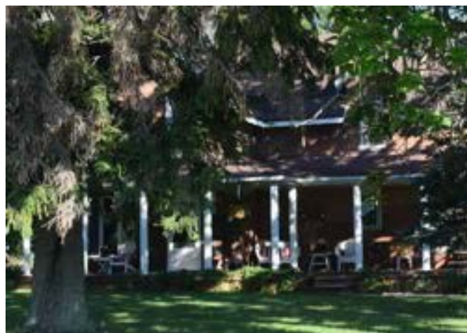
South (front) façade of house on property
