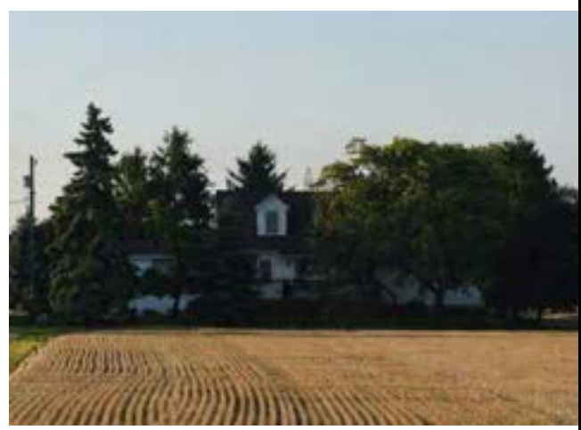
South (front) façade of house on property
