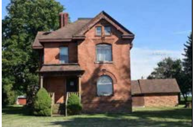
North (front) façade of house on property
