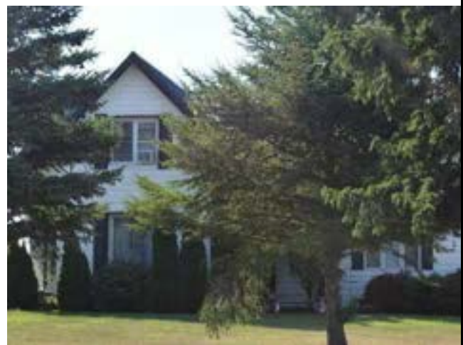
North (front) façade of house on property
