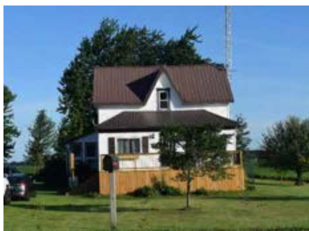
South (front) façade of house on property
