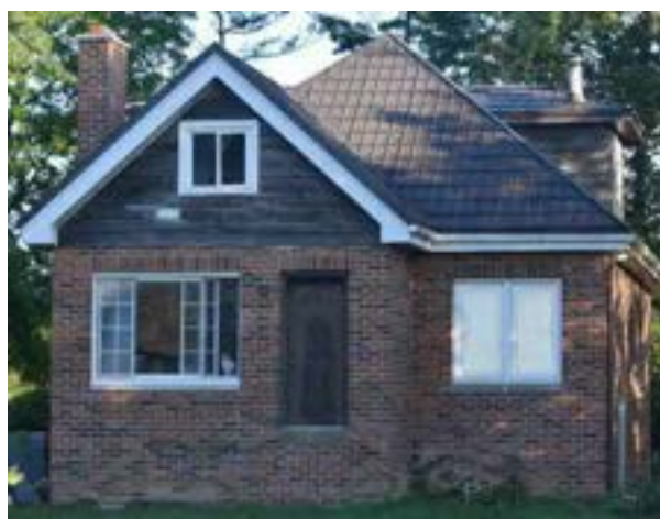
South (front) façade of house on property
