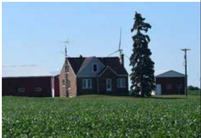
North (front) façade of house on property
