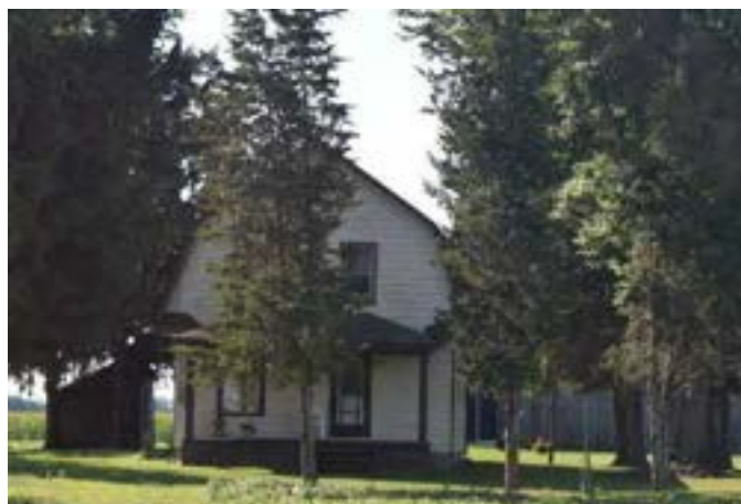
North (front) façade of house on property
