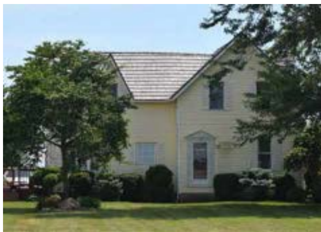
North (front) façade of house on property
