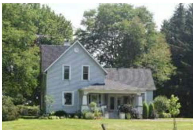
North (front) façade of house on property
