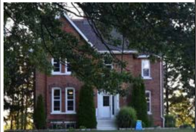
South (front) façade of house on property
