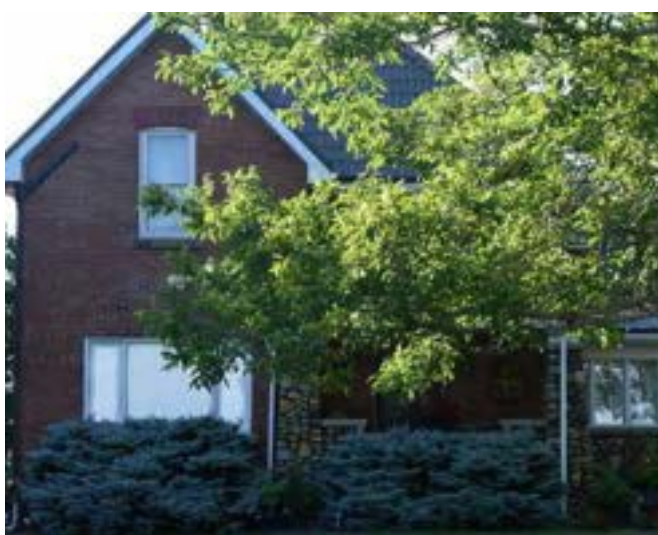
South (front) façade of house on property
