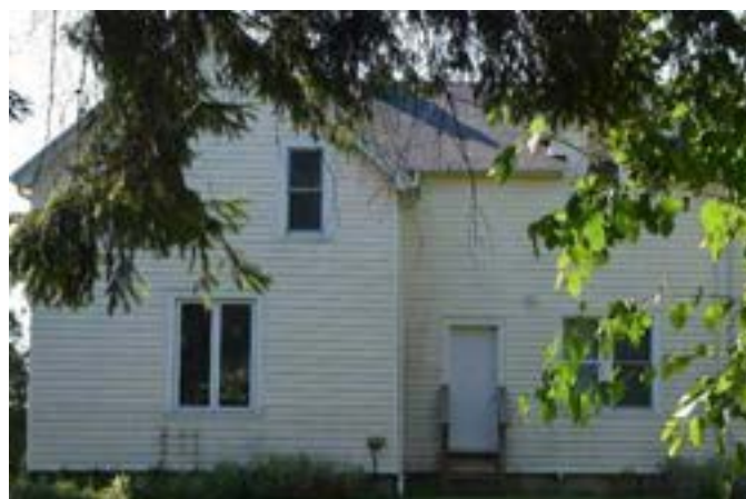
South (front) façade of house on property
