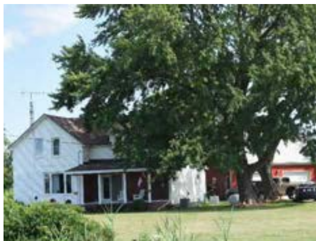
North (front) façade of house on property
