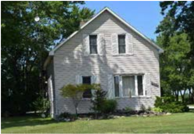
South (front) façade of house on property
