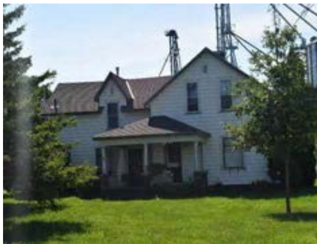
North (front) façade of house on property
