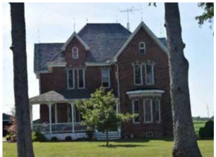
North (front) façade of house on property
