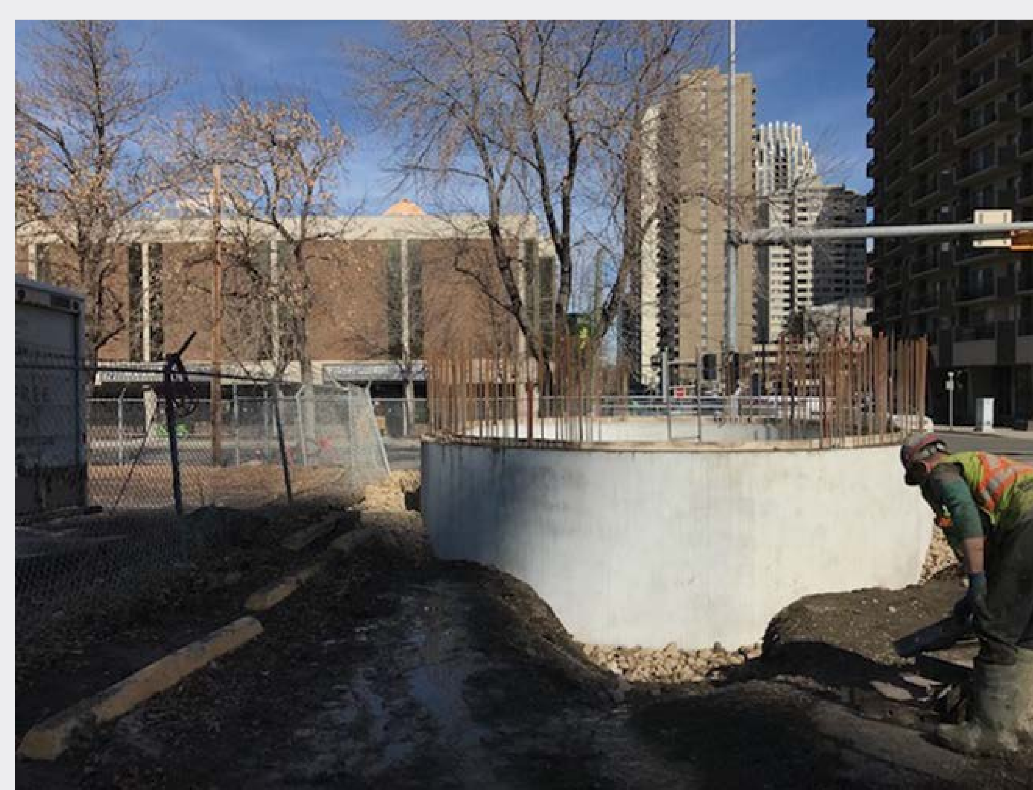
Example of shaft required for micro-tunneling construction
