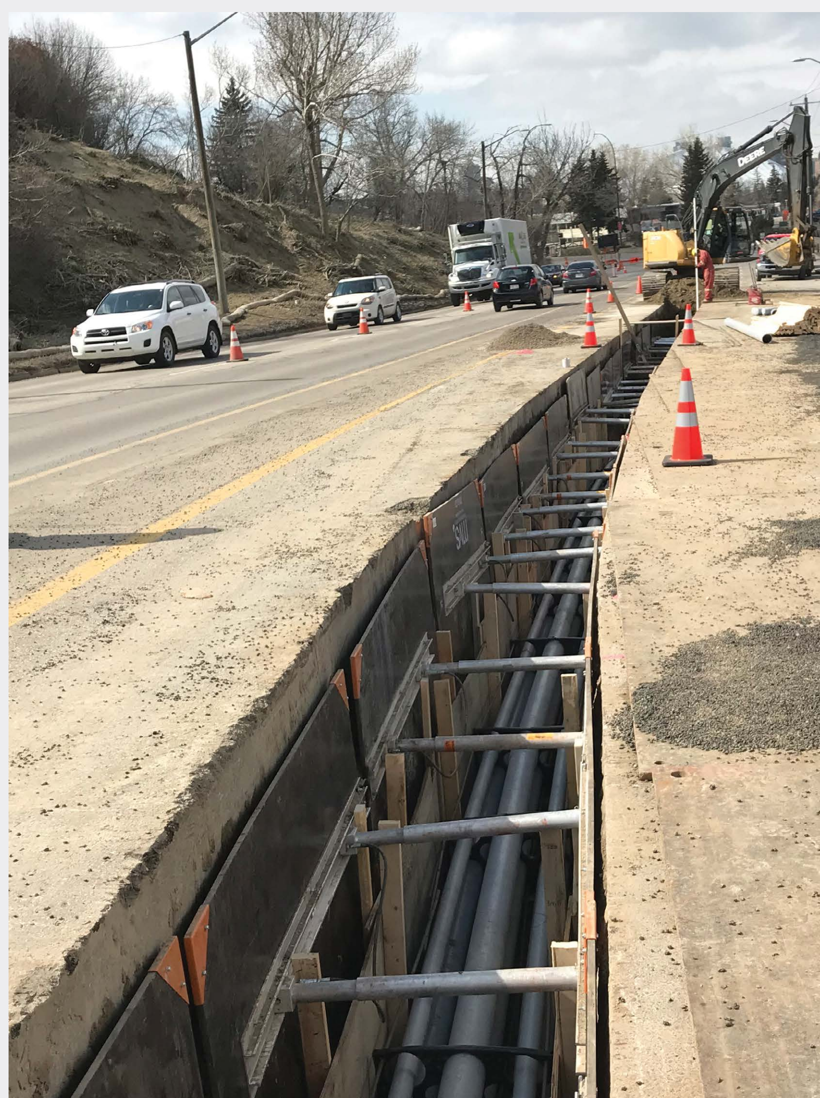
Example of open cut construction
