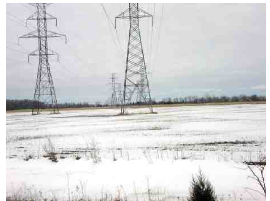
12 - Existing Hydro Corridor (looking west from Hwy 77)
