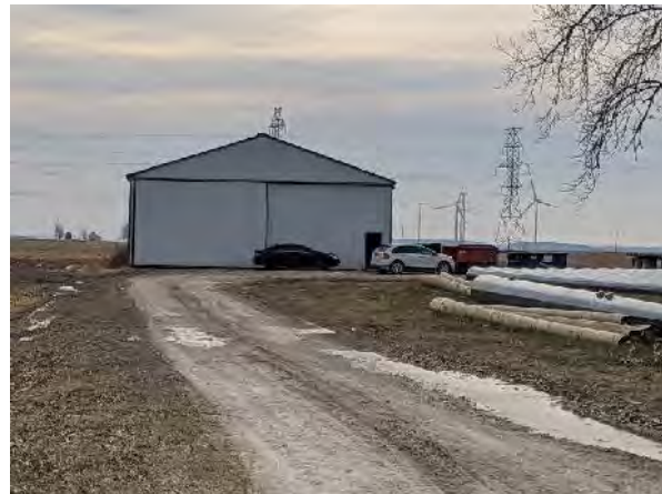
Plate 2: Photo of 3097 Middle Road showing new storage facility
