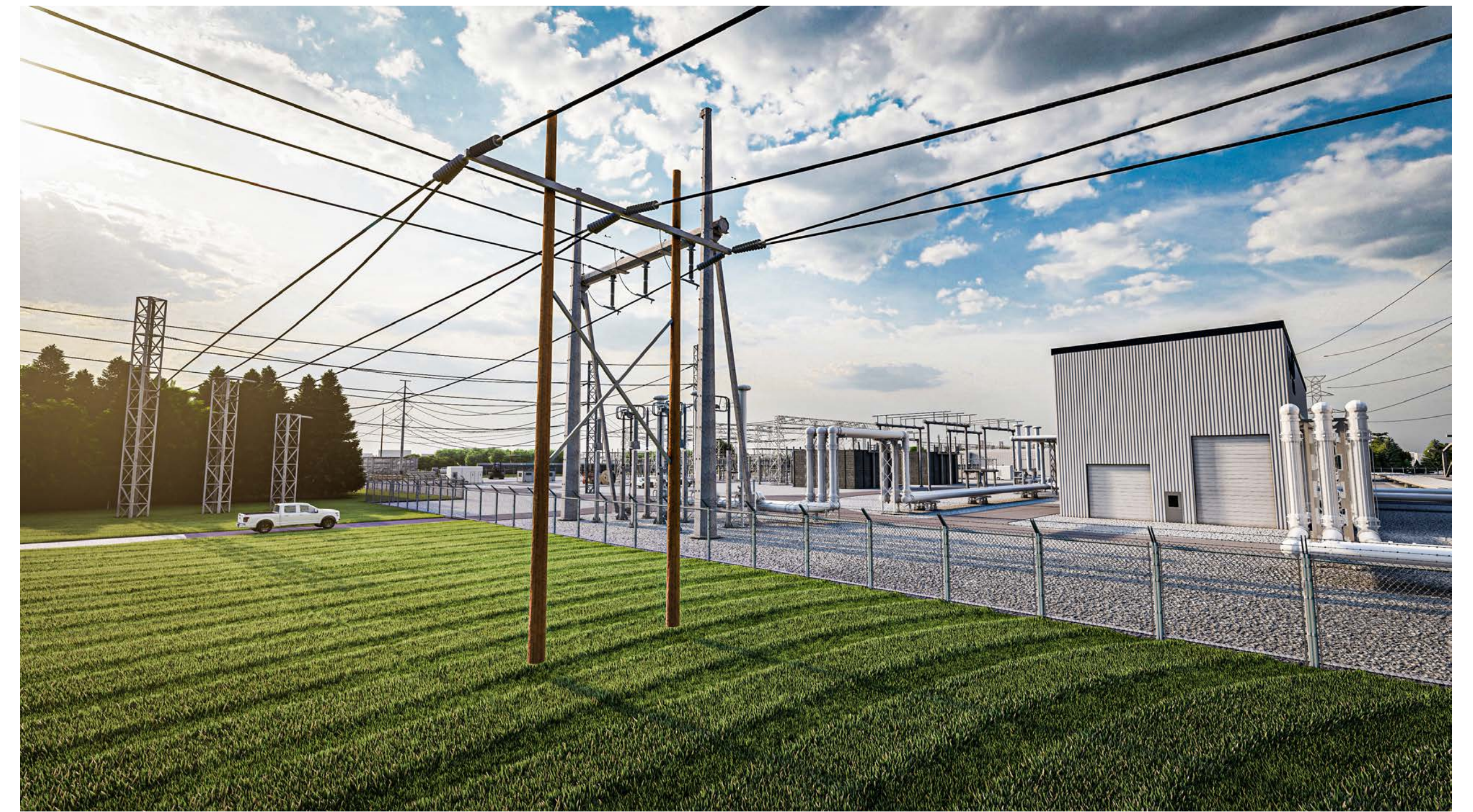
H-Frame Wood Structure
