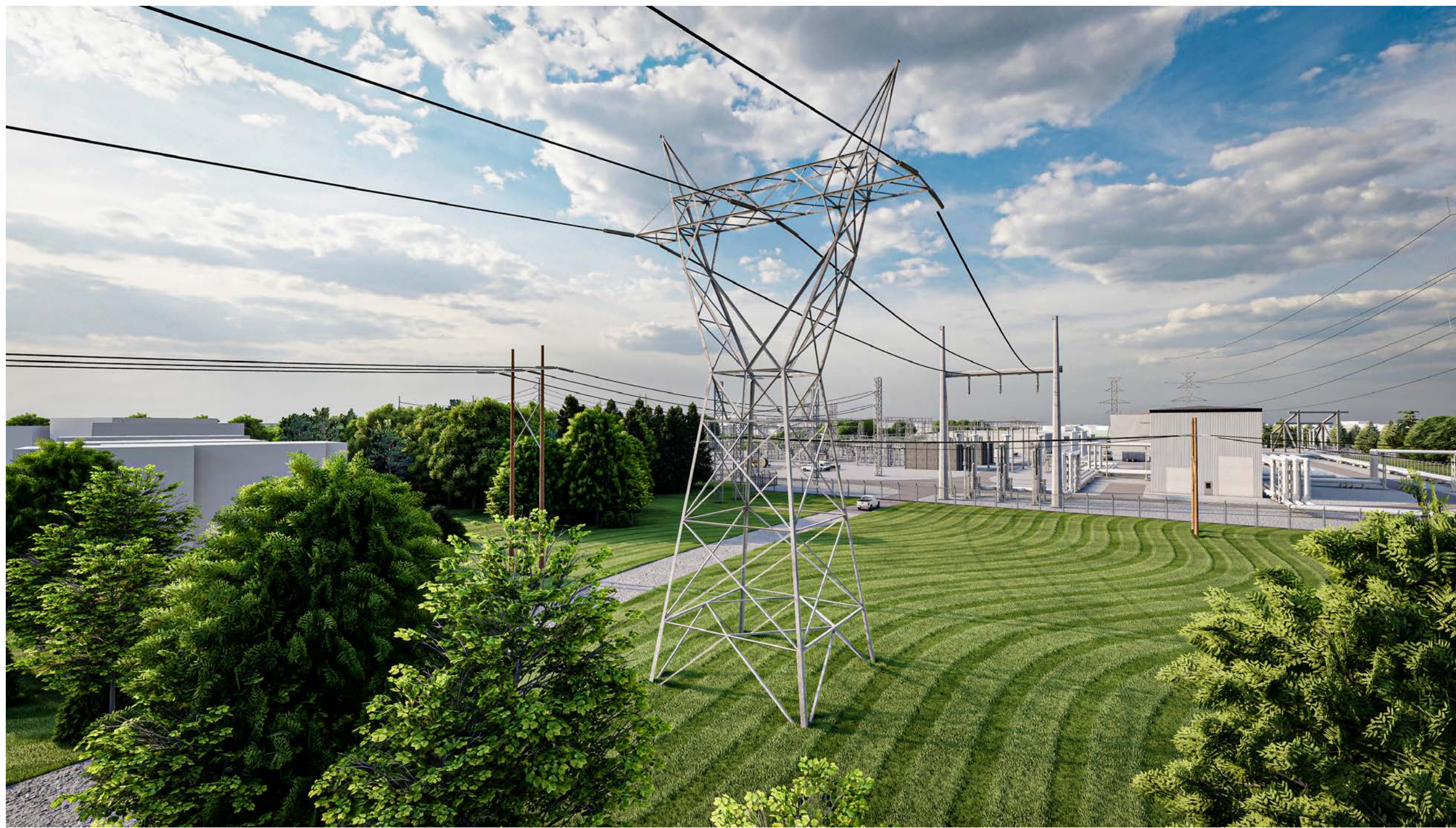
Lattice Steel Tower
