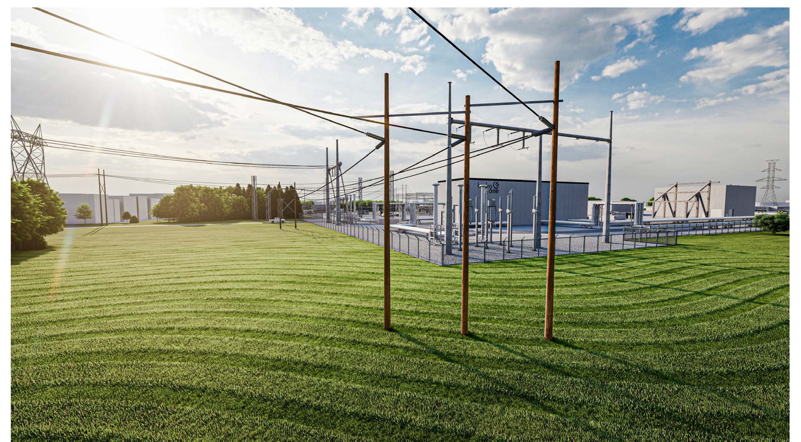
Dead End Wood Structure
