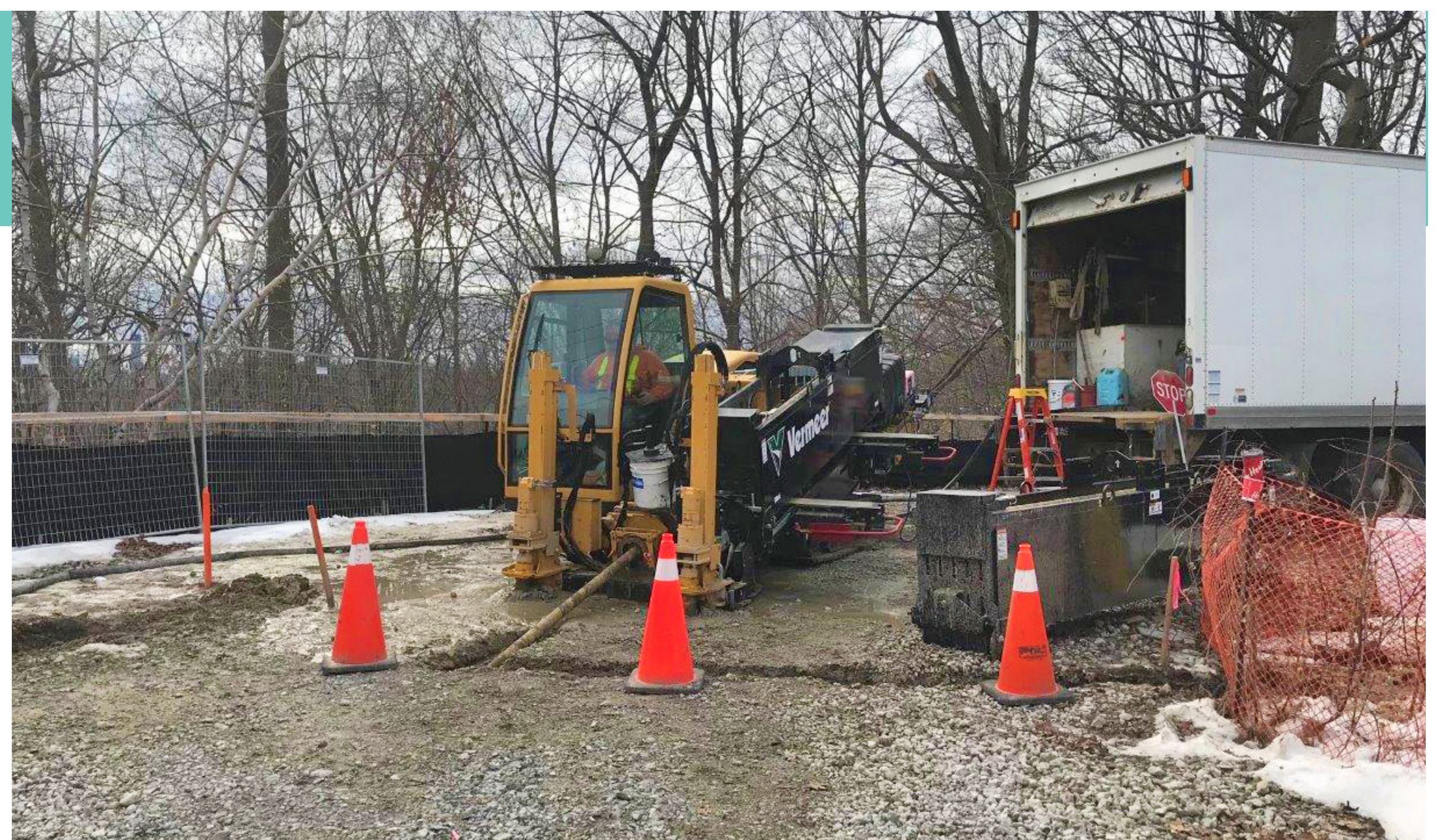
Example of directional drilling
