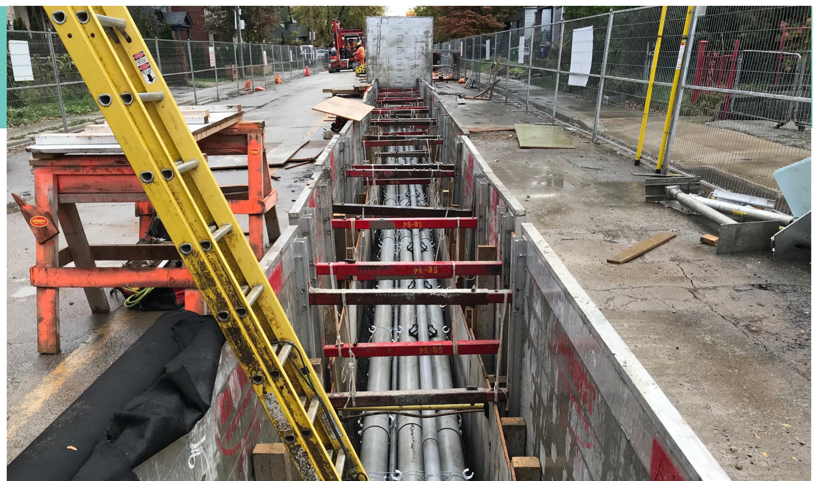
Example of open cut trenching
