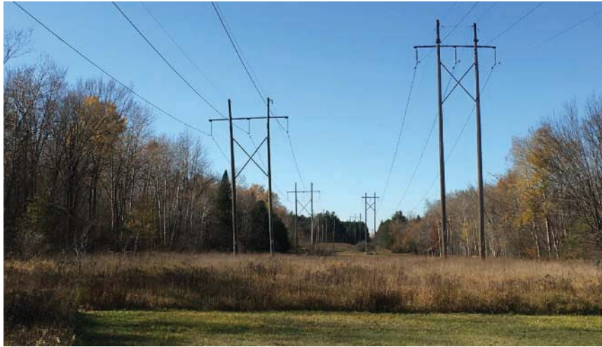
The existing structures are between 50-80 ft high
