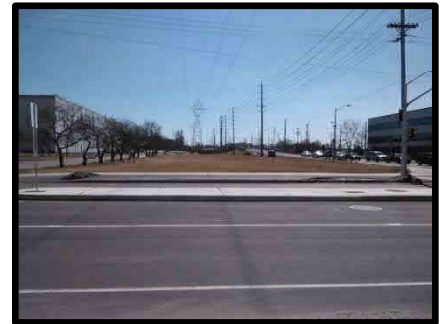
Coventry Road looking south
