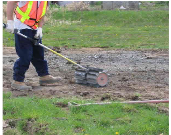
Remove remaining crushed stone
