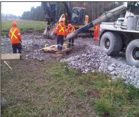
Pouring concrete for tower foundation
