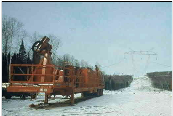
Pulling new conductor into position
