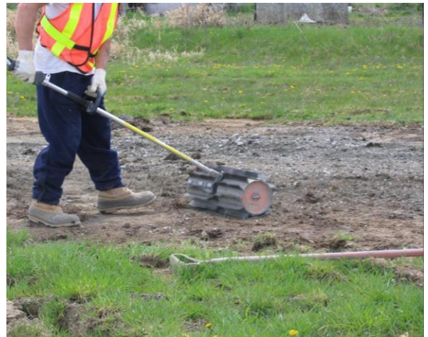
Remove remaining crushed stone
