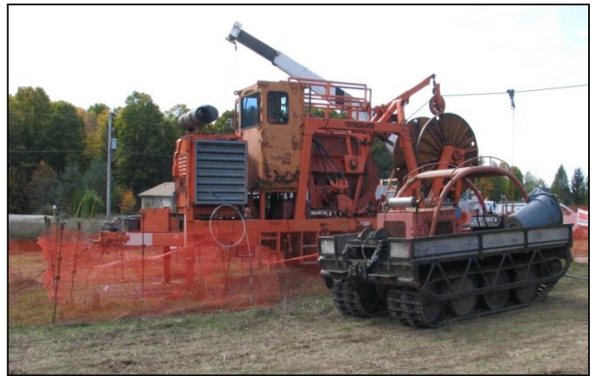
Set up laydown area
