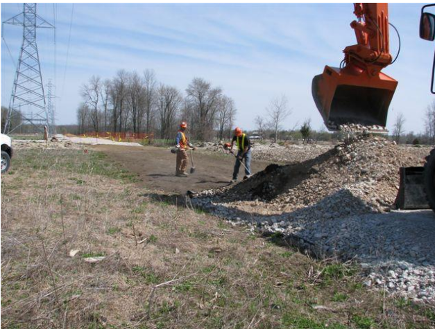
Remove temporary access road
