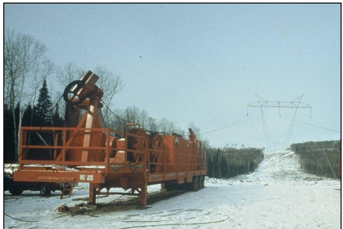
Pulling new conductor into position
