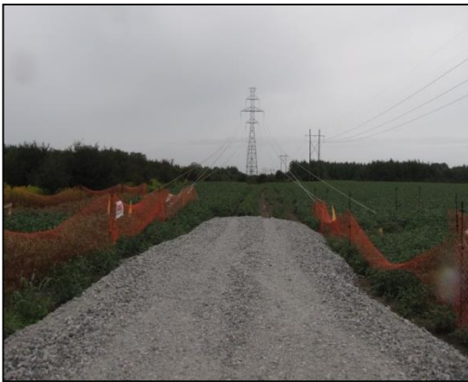
Temporary access road
