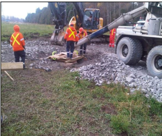
Pouring concrete for tower foundation
