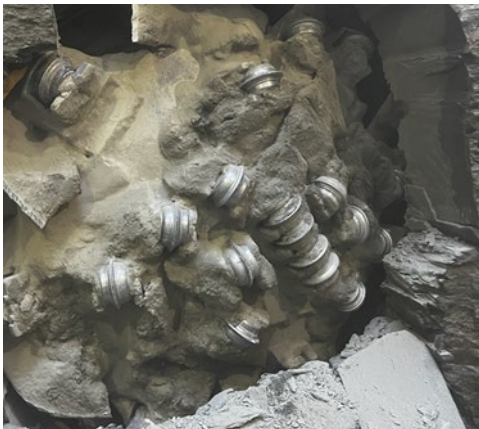
Front view of the tunnel boring machine within Terauley TS
