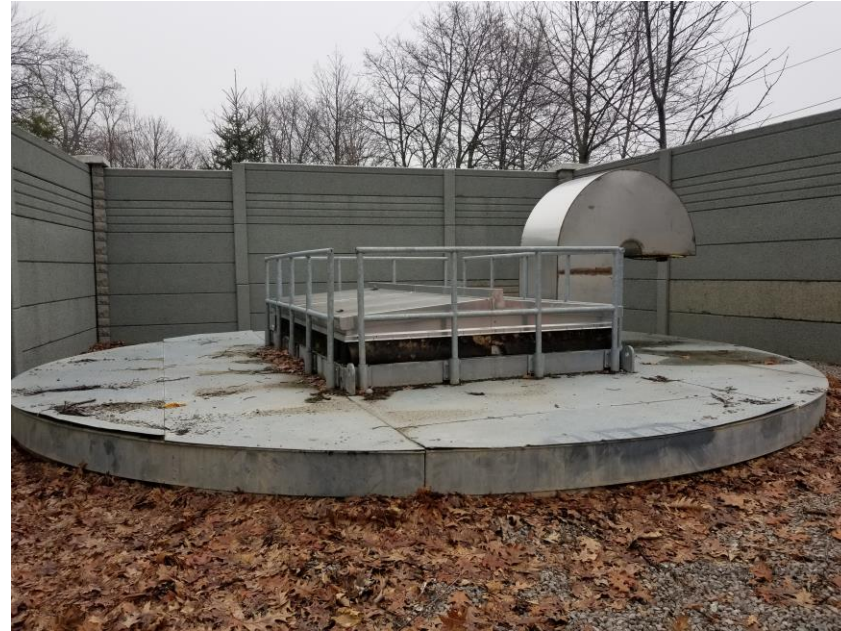
Example of a tunnel exit shaft
