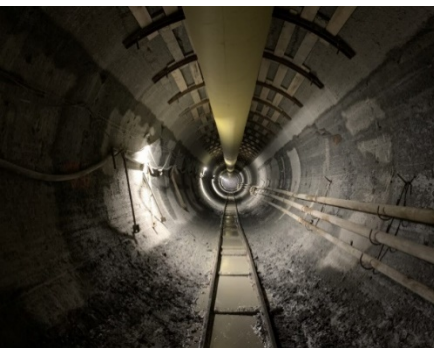
Photo of the new tunnel near the mid-point.
